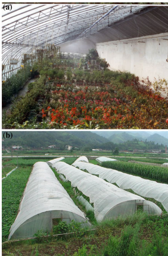
Fig. 12 Simple greenhouses a solar-heated earth-walled greenhouse, b arch-type plastic tunnel greenhouse. Photos Ziyong Huang and Guo (2010)
