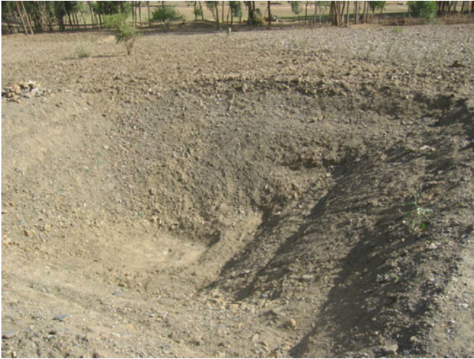
Fig. 8 Hard bedrock encounter at shallow depth. Location: Woreda Gulomekeda, Tabia Kileat. Photograph Gebremedhin Berhane
