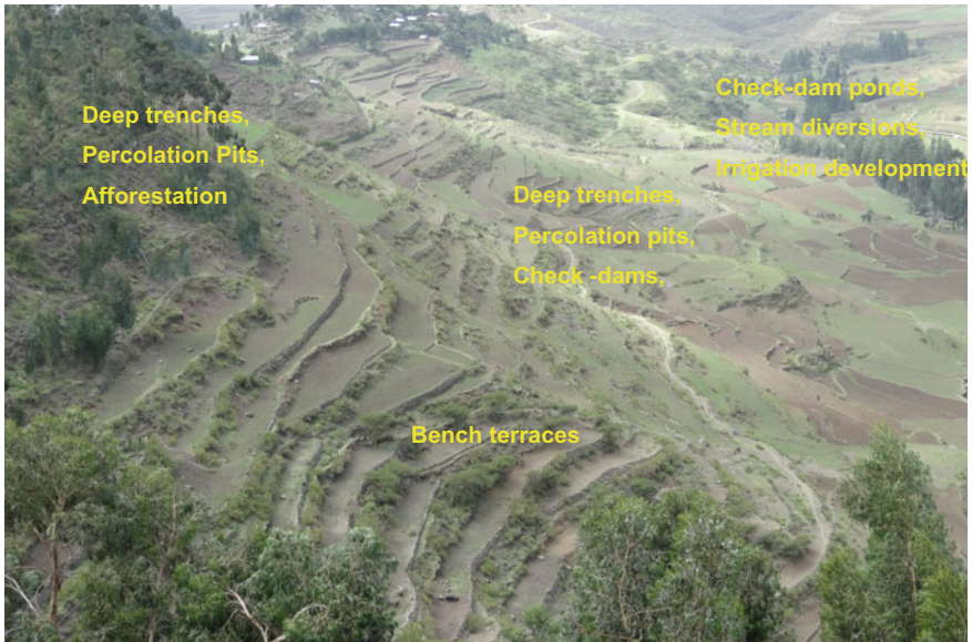
Fig. 2 An overview of implementation of complementary/linked LRWH technologies considering site-specific conditions and the landscape continuum in Tigray, Ethiopia. Photograph Kifle Woldearegay
