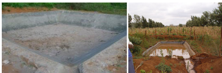
Fig. 3 Attempts to control seepage (lining with masonry works and plastic). Photographs Stephen Ngigi
