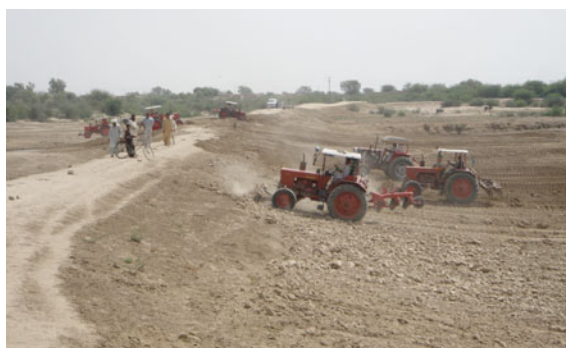
Fig. 3 Soil bunds preparation in Dera Ismail Khan, Pakistan. Photograph MetaMeta
