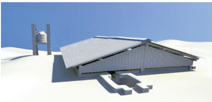
Fig. 4 A runoff pond covered with iron sheet. Source Pixiniti Studios
