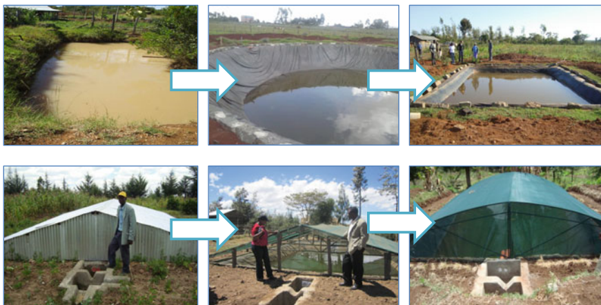
Fig. 6 Evolution of water losses (seepage and evaporation) control measures. Photographs Stephen Ngigi
