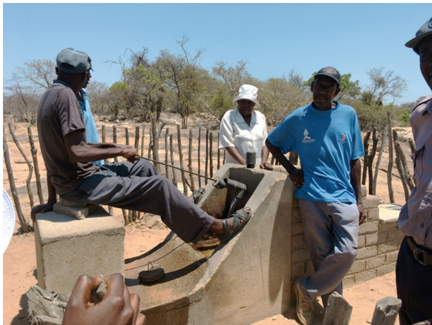
Fig. 10 Simple manual pumping to extract water from a sand dam in Umzingwane, Zimbabwe. Photograph Rumbidzai Nyawasha
