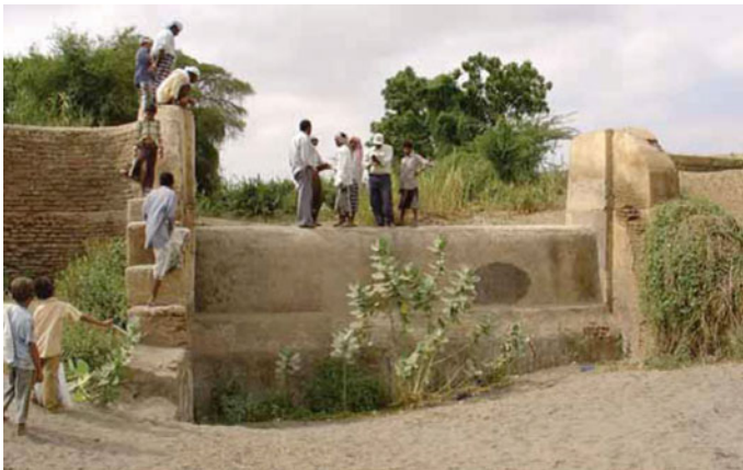
Fig. 6 Stepped drop structure, Wadi Zabid, Yemen. Photograph MetaMeta
