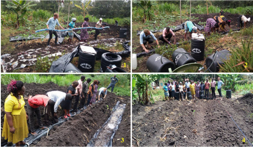
Fig. 7 Step-by-step GRP construction phases. Photos Lucas Zahl
