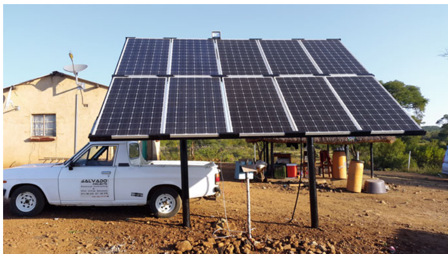
Fig. 8 Solar power unit used to pump water for irrigation. Photograph Menas Wuta
