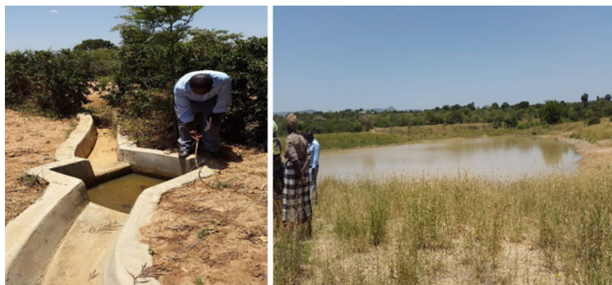
Fig. 4 Roadside diversion ditches can be used to collect runoff water which can collect in roadside ponds. Photograph Means Wuta
