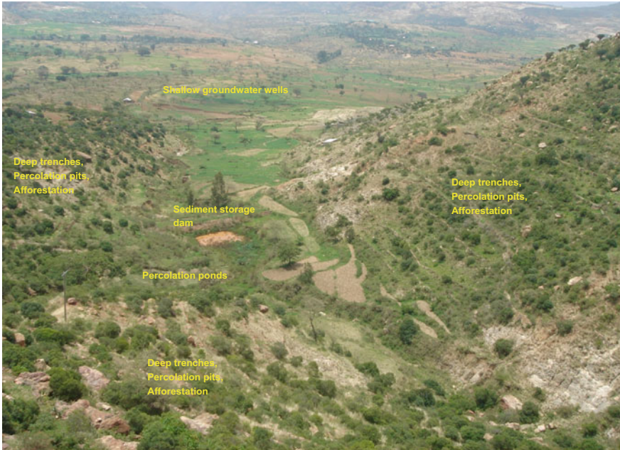
Fig. 7 View of some of the LRWH technologies implemented in Sero watershed, Tigray, Ethiopia. Photograph Kifle Woldearegay
