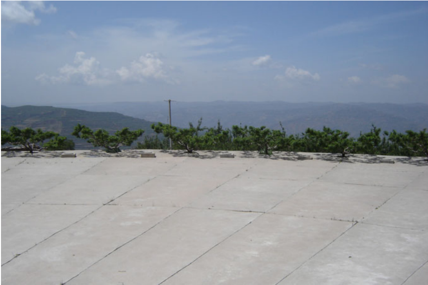
Fig. 4 Concrete-lined catchment for irrigating orchards in Qin'an County. Photo Zhu (2003)
