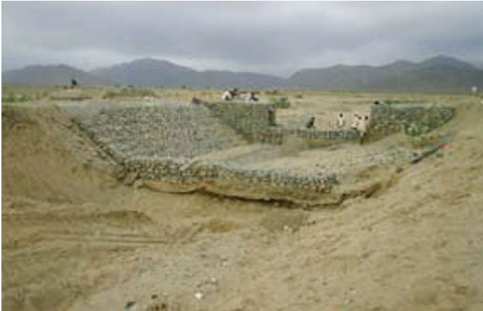
Fig. 7 Flow division and channel bed stabilizer. Photograph MetaMeta
