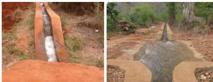
Fig. 5 Improved, lined irrigation canals to transfer water with minimum conveyance losses and shorter time from dam reservoir to field, Bangala, Tanzania. Photographs Sokoine University of Agriculture, Tanzania
