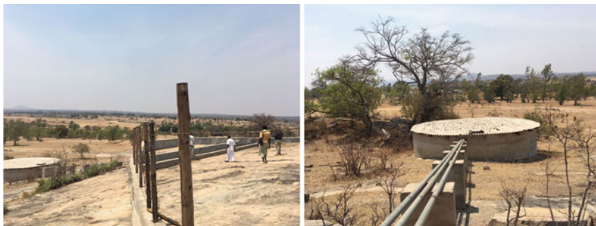
Fig. 7 Rock catchment and brick water storage tank in Mutoko, Zimbabwe. Photograph Menas Wuta
