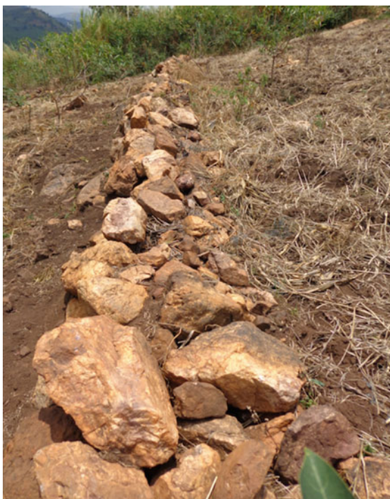
Fig. 3 A newly constructed stone bund. Photo James W. Kisekka
