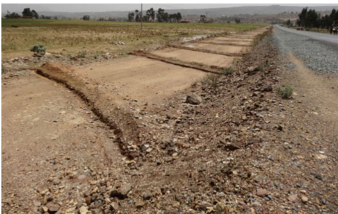
Fig. 2 Water spreading from road surface to farmlands in Tigray, Ethiopia. Photograph Kifle Woldearegay
