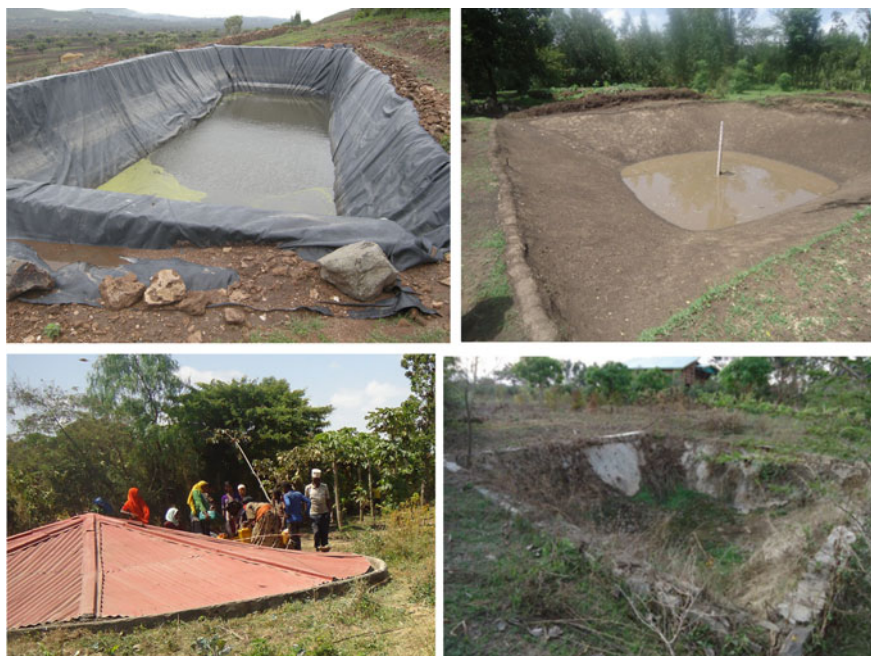
Fig. 3 Household ponds in Alaba, Ethiopia: a trapezoidal pond lined with geo-membrane. Plastic for seepage control (upper left); a recently established earthen pond (upper right); a concrete pond with corrugated iron cover to reduce evaporation losses (lower left) and a non-functioning concrete pond without cover (lower right). Photographs Adana Abebe Awass and Hussen Abdela
