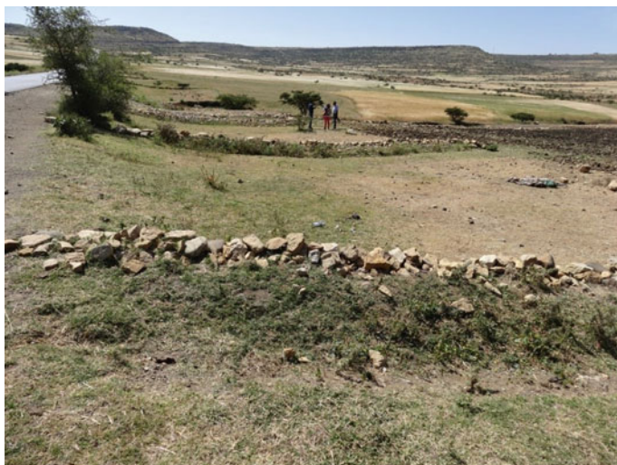
Fig. 8 Diverting roadside runoff into farmlands as part of moisture conservation in Kiken area (along Mekelle-Wukro road), Tigray, Ethiopia. Source Kifle Woldearegay
