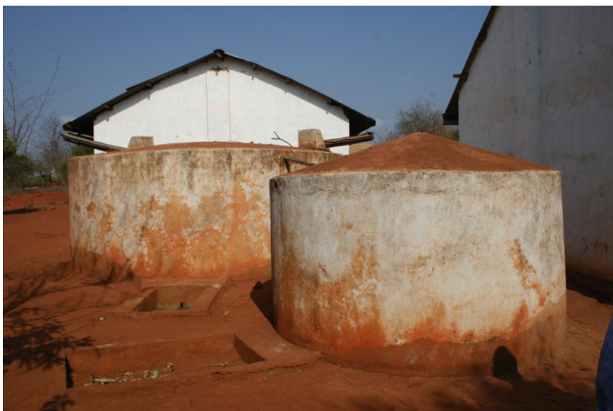
Fig. 4 Roof catchment system with ferro-cement tanks. Photograph Josep de Trincheria Gomez
