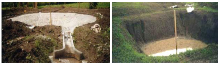
Fig. 2 Monitoring water losses from a lined and unlined farm ponds. Photographs Stephen Ngigi
