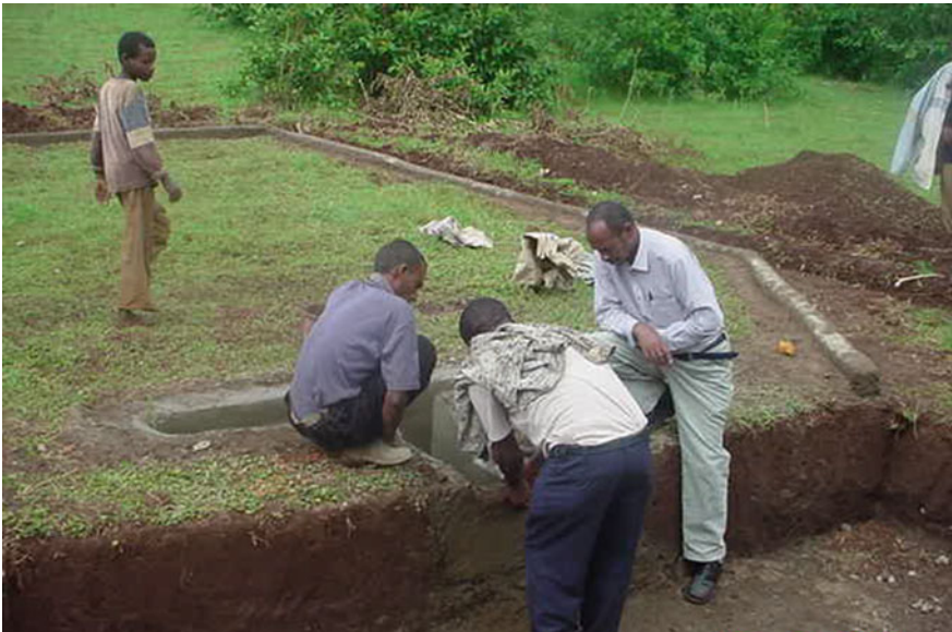
Fig. 4 Construction of grass collection catchment (GCT). Photograph Alemayehu Haddis
