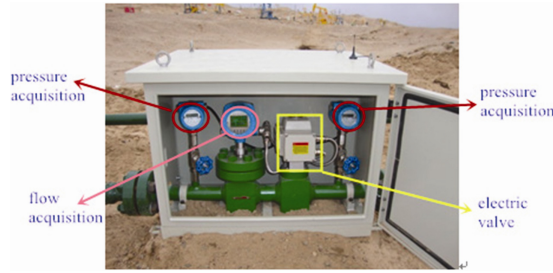
Fig. 2. Skid-mounted structure of flow automatic control instrument
