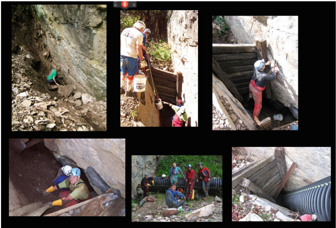
Fig. 10.33 Wildcat Entrance is critical as an easy access to both the Culverson and McLaughlin parts of the cave system. Unfortunately, the entrance was not stable and frost shatter caused the scree slope from the escarpment above to fill and collapse the entrance. To remedy the situation, the unstable area was enlarged, shored, and a 20-foot plastic
