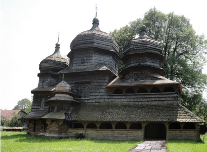
Fig. 4.1 Domes from logs of the Orthodox church in Drohobych, photograph by the author
