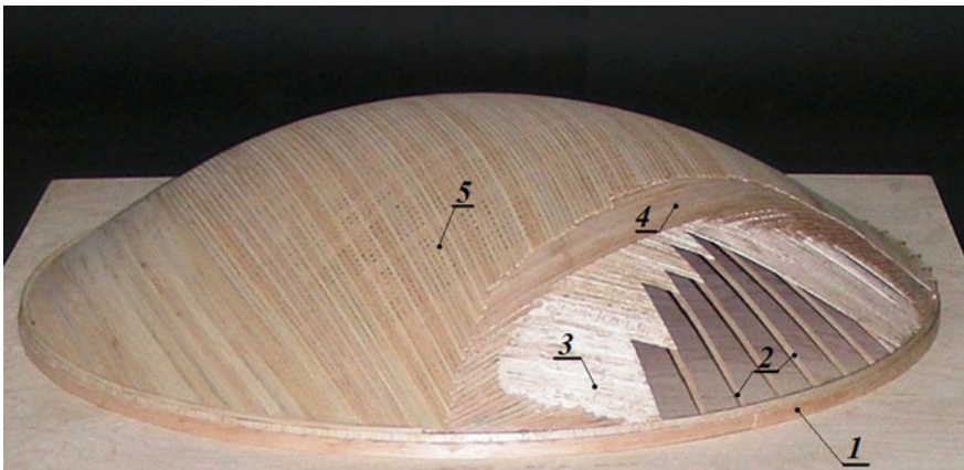
Fig. 6.4 Model of a shell dome of a 17.5 m diameter at a scale 1:30 according to [3]
