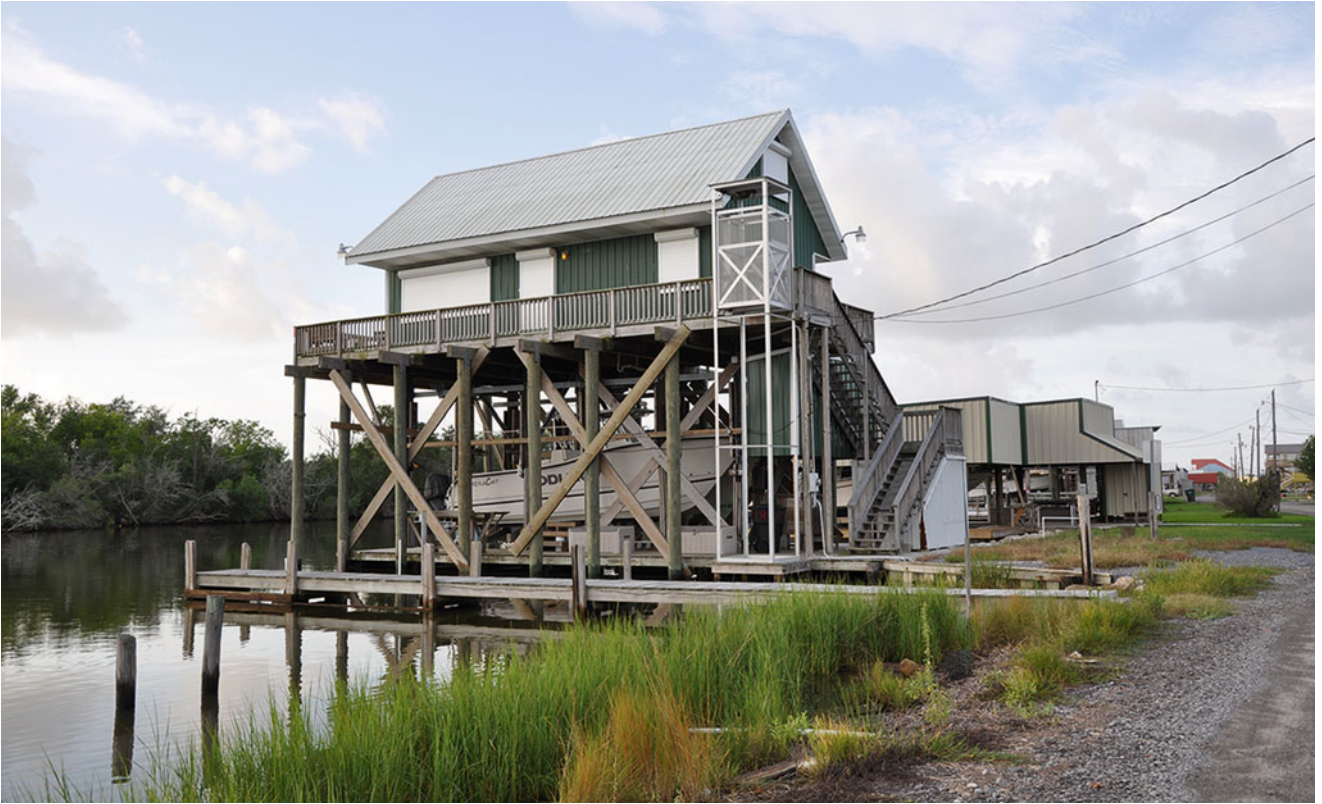
Fig. 13 Elevated home with elevator in Cocodrie, LA (Credit: LSU Coastal Sustainability Studio)
