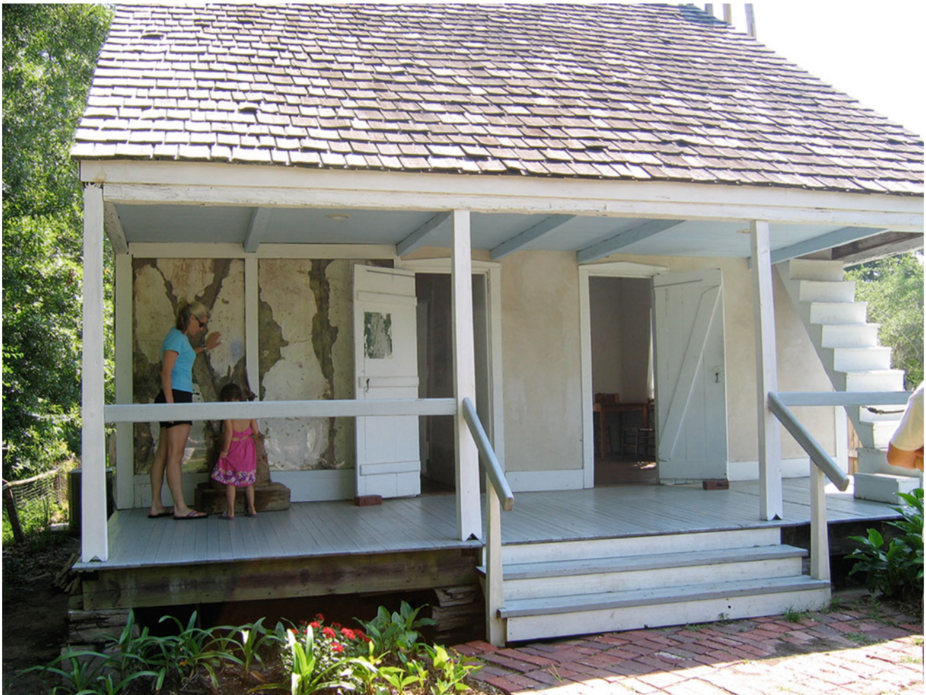
Fig. 16 Traditional Louisiana Cypress Timber construction in Lafayette, LA (Credit: Jori Erdman, LSU School of Architecture)
