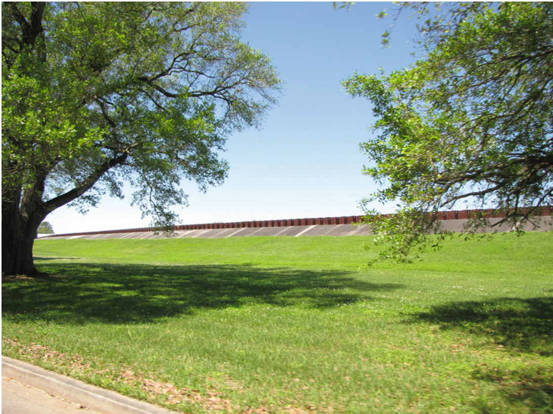
Fig. 9 The levee along Orleans Avenue Outfall Canal (Credit: Giovanni Coakley)
