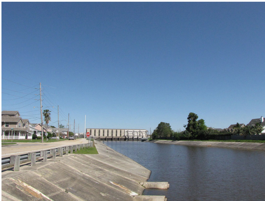
Fig. 10 Pump station in Metarie (Credit: Giovanni Coakley)
