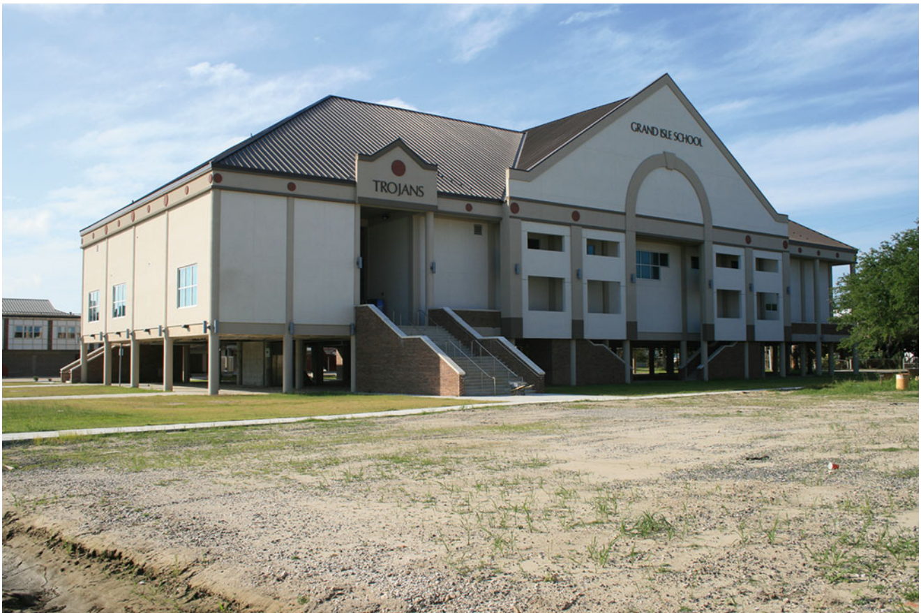
Fig. 25 Completed in 2011, the gymnasium of Grand Isle School is elevated approximately 12 ft above grade and built to withstand 150 mph winds and the harsh saltwater environment of Grand Isle, LA (Credit: LSU Coastal Sustainability Studio)
