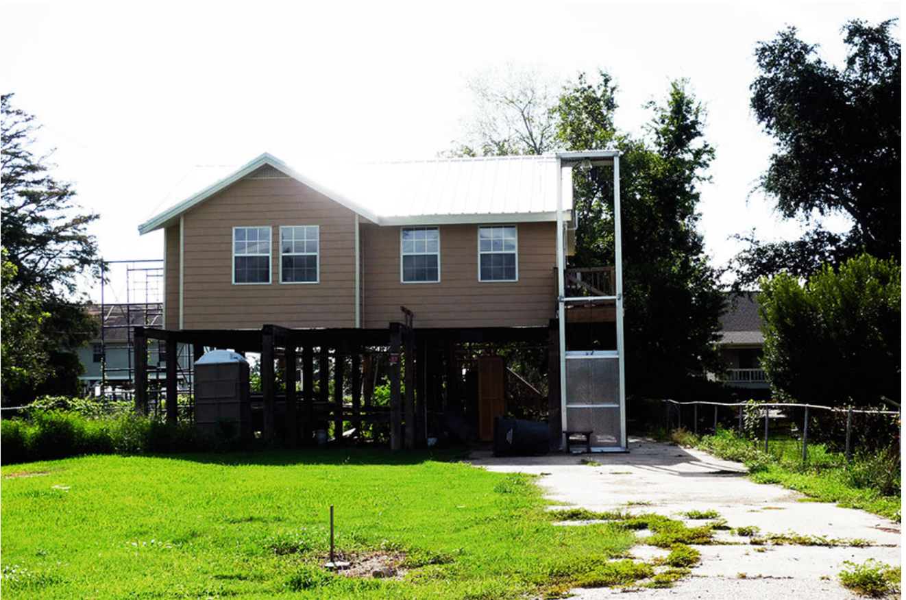
Fig. 14 Elevated home with elevator in Dulac, LA (Credit: LSU Coastal Sustainability Studio)
