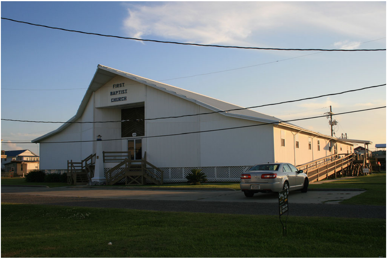
Fig. 24 The original slab-on-grade structure of First Baptist Church in Grand Isle, LA is now elevated on piers (Credit: LSU Coastal Sustainability Studio)
