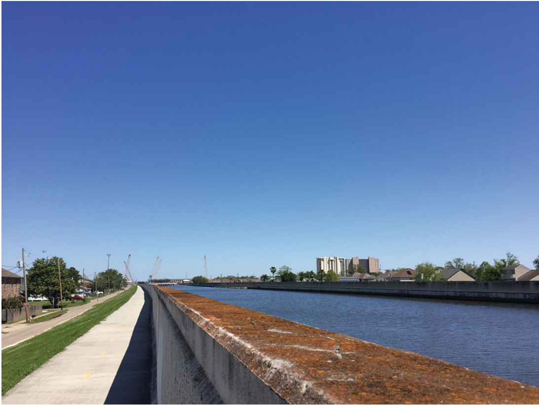
Fig. 8 The levee along 17th Street Outfall Canal (Credit: Christopher James)
