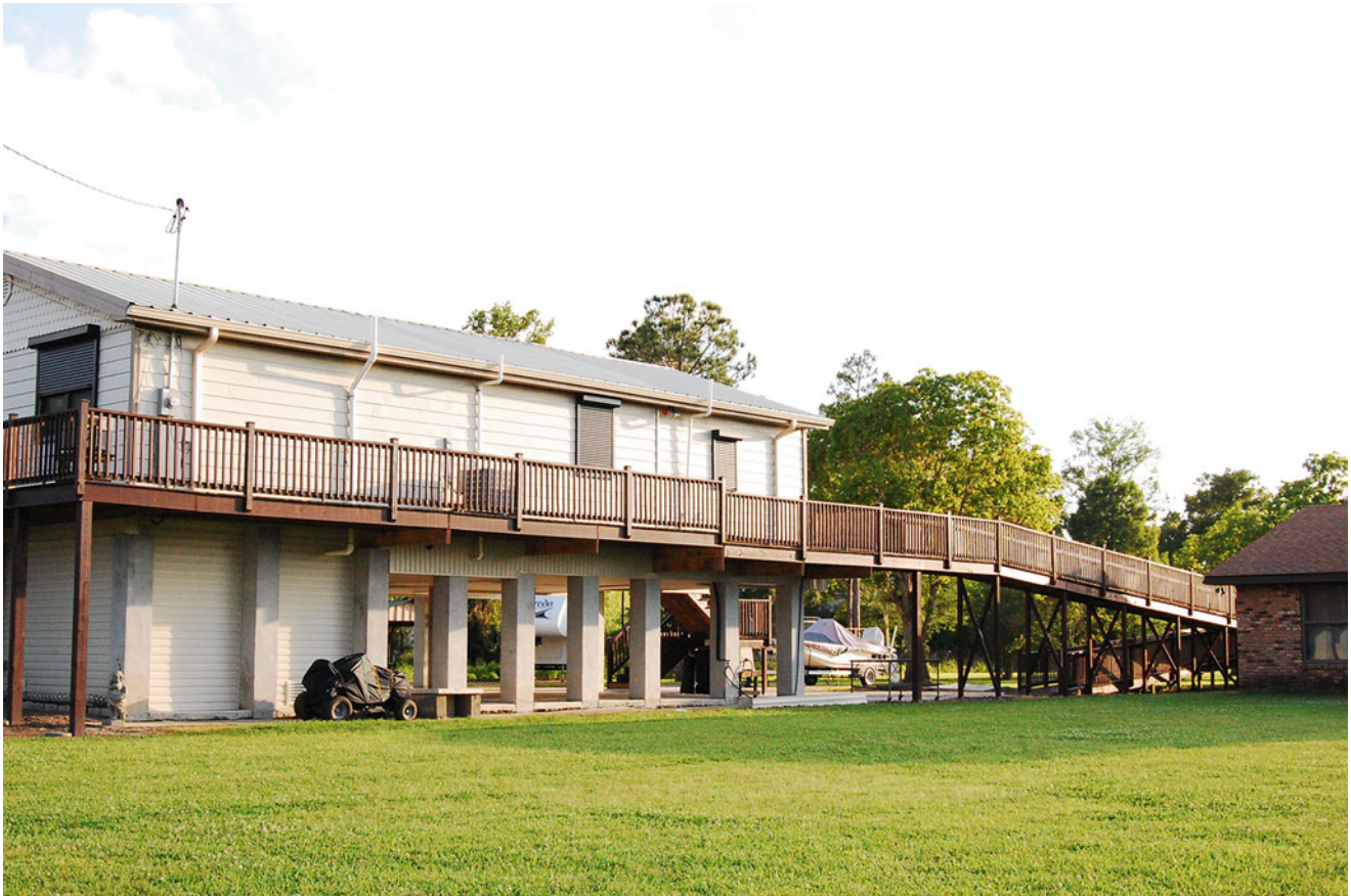
Fig. 10 Elevated home in Lafitte, LA with ramped access (Credit: LSU Coastal Sustainability Studio)
