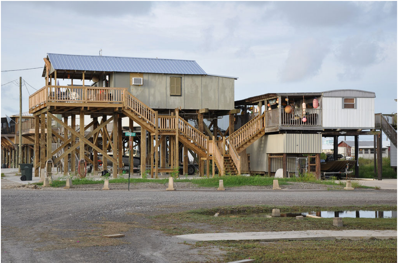
Fig. 7 Elevated homes with shared staircase in Cocodrie, LA (Credit: LSU Coastal Sustainability Studio)
