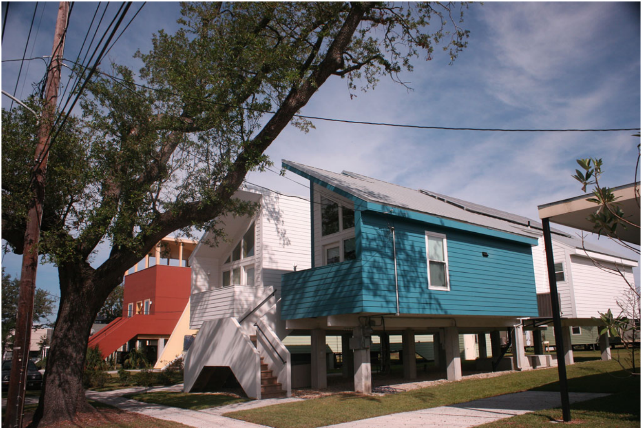
Fig. 27 Elevated homes in the Lower Ninth Ward of New Orleans (credit: Drew from Zhrodague, CC by 2.0, https://www.flickr.com/photos/drewzhrodague/8123959293/in/photolist-dnTq4F-8LeiR-dnTw2d-dnTyEG-dnTqFZ-8Le5g-dnTuYa-dnTxc-6lhgs1-8Le5W-8Le4W-72Kkfq-dnTv8r-dnTv2x-dnTqMc-8LdUm-8LekS-dnTxVX-8Leoh-dnTr6e-8Ld
