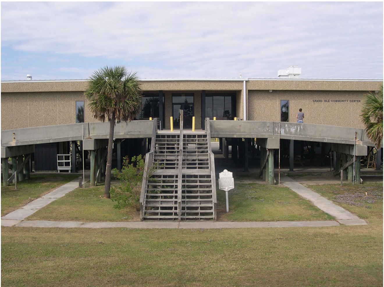
Fig. 26 The elevated community center in Grand Isle, LA (Credit: LSU Coastal Sustainability Studio)
