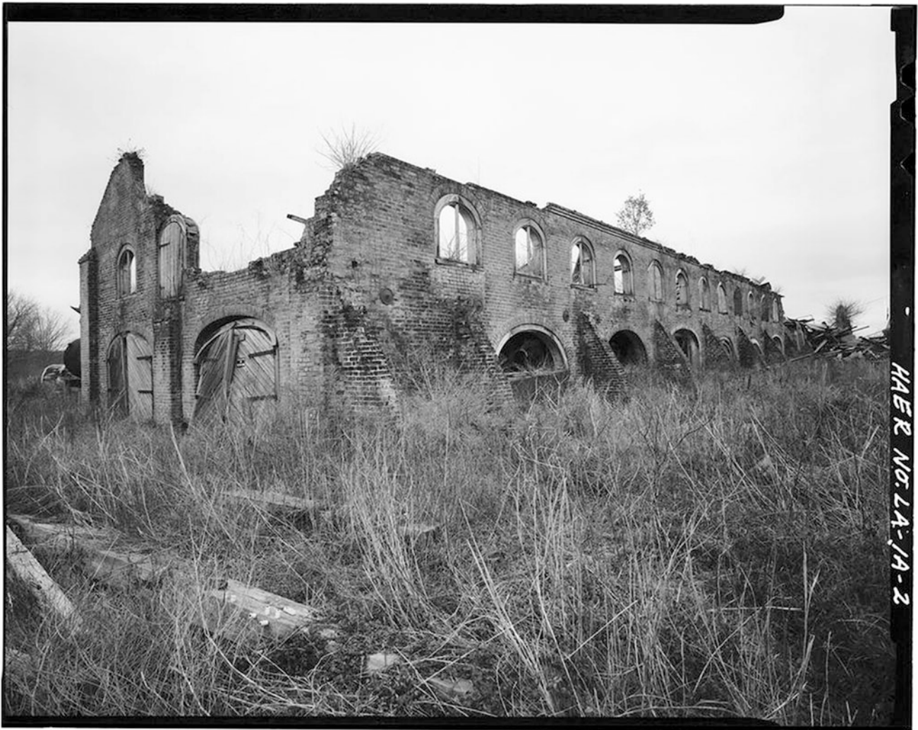
Fig. 18 Brick construction of the Laurel Valley Sugar Plantation in Thibodaux, LA (Credit: Library of Congress Prints and Photographs Division Washington, DC. 20540 USA – HAER LA,29-THIB,1A—2 – http://www.loc.gov/pictures/item/la0195.photos.072549p/ )
