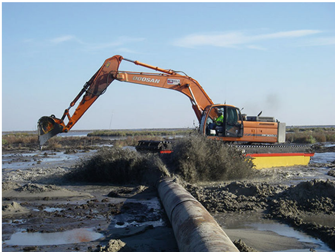
Fig. 15 Sediment from the Mississippi River delivered to marsh-building projects by the Coastal Wetlands Planning, Protection, and Restoration Act (Credit: CWPPRA – https://lacoast.gov/new/About/ )
