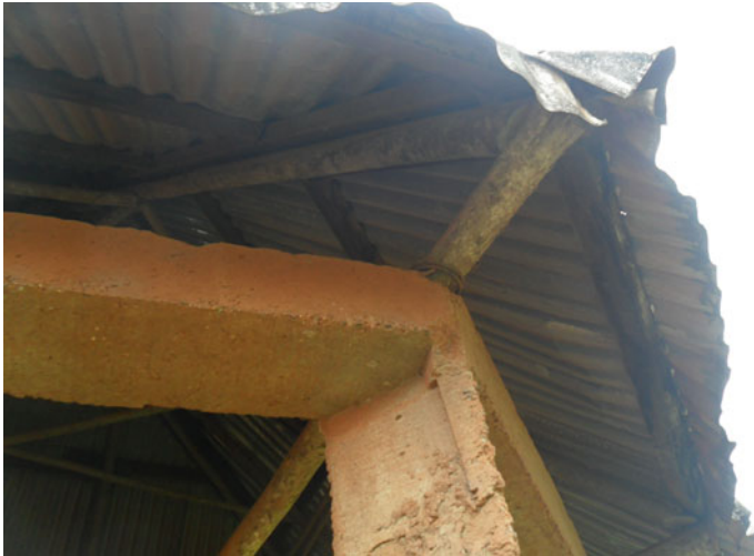
Fig. 5.5 Wooden poles used as wall plates, rafters and purlins
