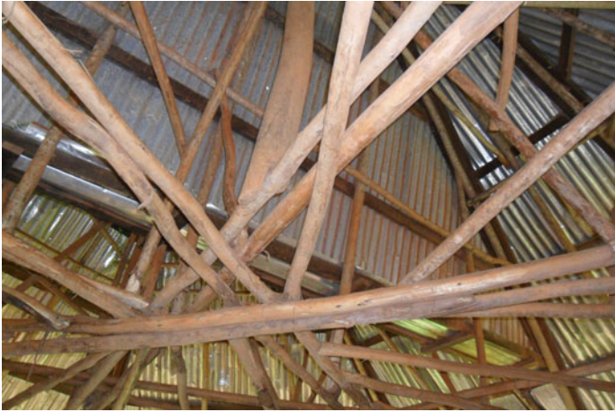
Fig. 5.6 Wooden posts and poles used as rafters
