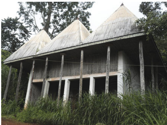
Fig. 9.4 Wooden poles used as long columns in a building
