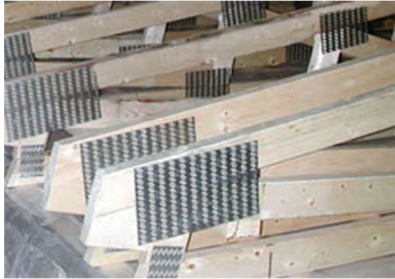
Fig. 12.5 Truss metal plates
