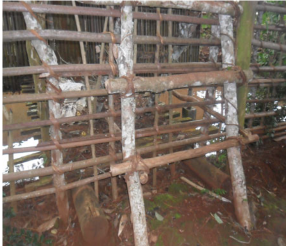
Fig. 9.2 Wooden posts used as short columns in fencing
