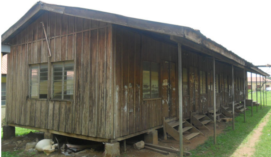
Fig. 1.3 A wood-framed building on concrete pile foundation
