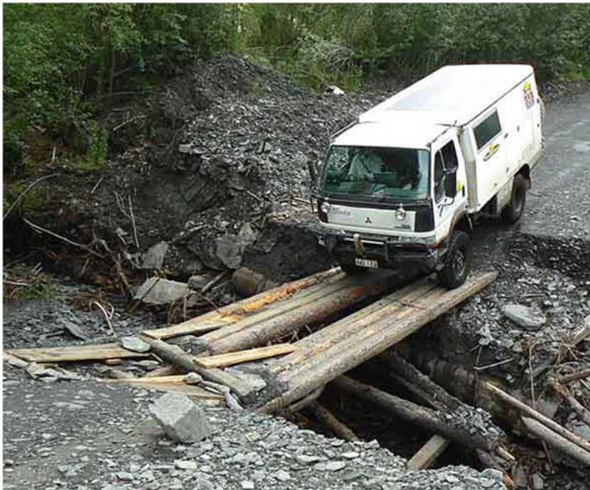
Fig. 13.1 a A single log bridge. b A multiple-log bridge
