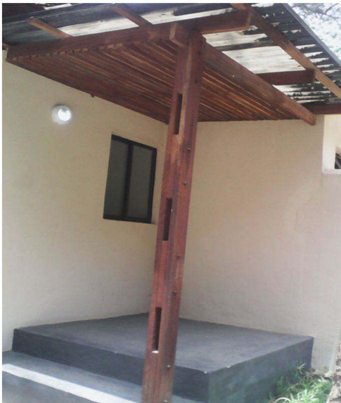
Fig. 10.1 A Spaced column
