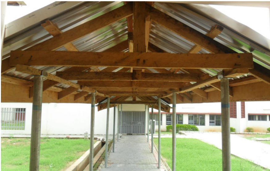
Fig. 1.1 Wooden rafter installation in a walkway
