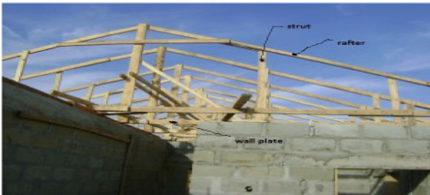
Fig. 12.2 A wooden truss installation in progress
