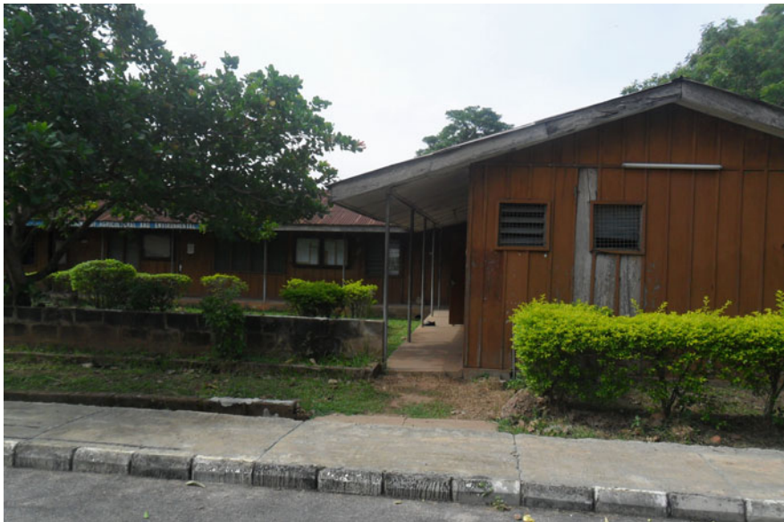
Fig. 1.4 A wood-framed building on sandcrete block foundation
