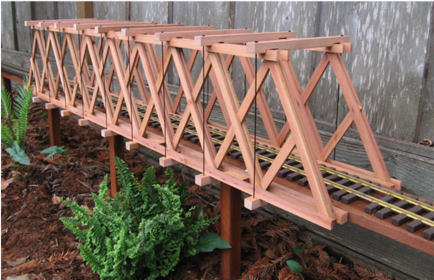
Fig. 13.4 a A typical wooden truss bridge. b A wooden truss bridge with iron rods as tension members
