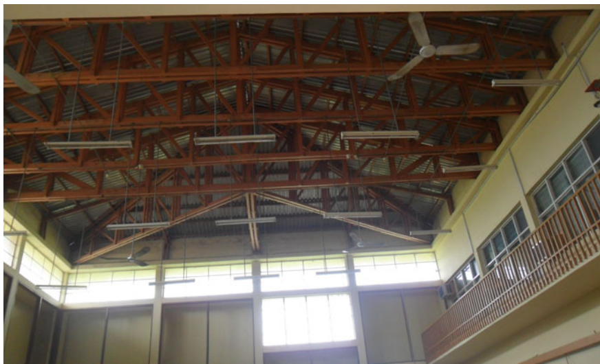
Fig. 1.2 Wooden truss installation in a workshop
