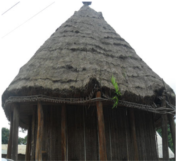
Fig. 5.3 Logs used as columns in a rural residential building
