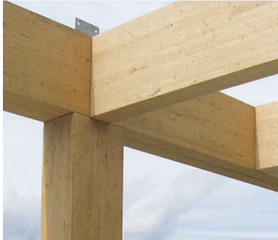
Fig. 8.8 A wooden bearing support for a set of wooden beams
