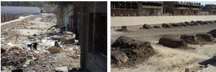
Fig. 2 During the excavation works and the foundations of the found Sphinxes
