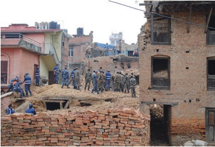
Fig. 1.1 Efforts post-earthquake to help affected people and to assess damage (Source: NSET)
