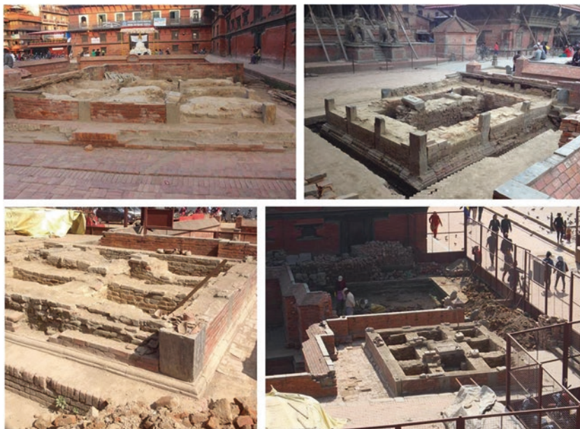
Fig. 10.3 Post-disaster stages of subsurface interventions at the Mani Mandapa, Patan. The southern pavilion, with soil fills intact post-earthquake, November 2015 ( top left ). Clearance of soil fills in the southern pavilion, May 2016 ( top right ). Soil removed from the northern pavilion, with ceramics present within the soil, February 2017 ( bottom left ). View to the south showing complete removal of foundations of the southern pavilion and surviving brick foundations of the northern pavilion after removal of soil fills, February 2017 ( bottom right )
