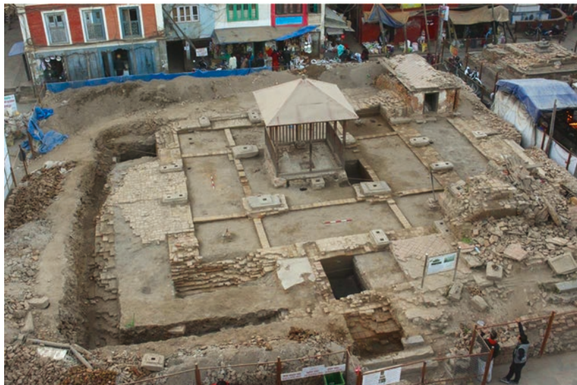
Fig. 10.12 Nine-celled mandala layout formed at the Kasthamandap by foundation wall, cross-walls and brick piers
