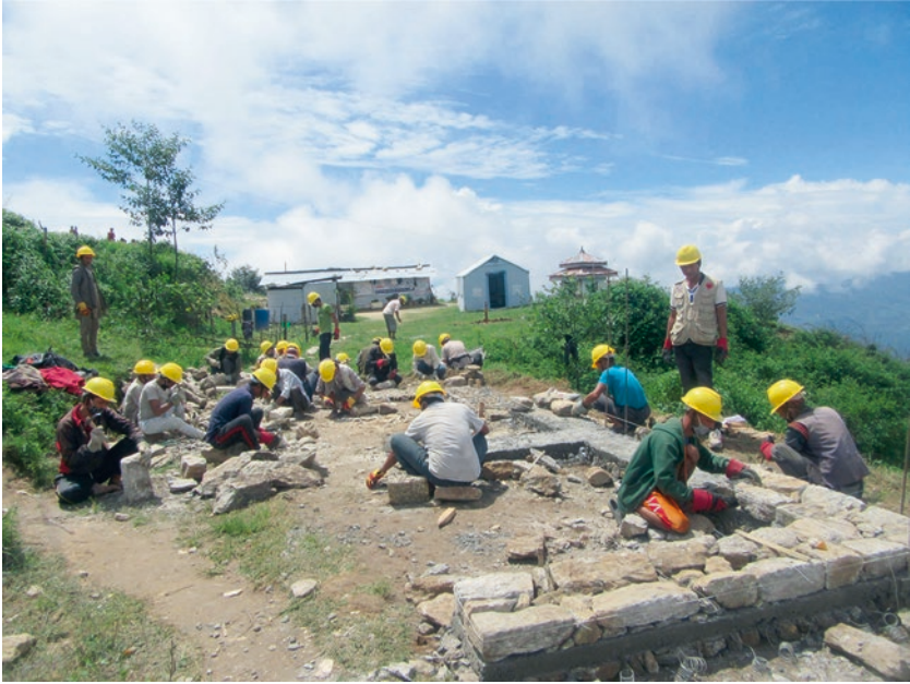
Fig. 2.3 NSET training local masons (Source: NSET)
