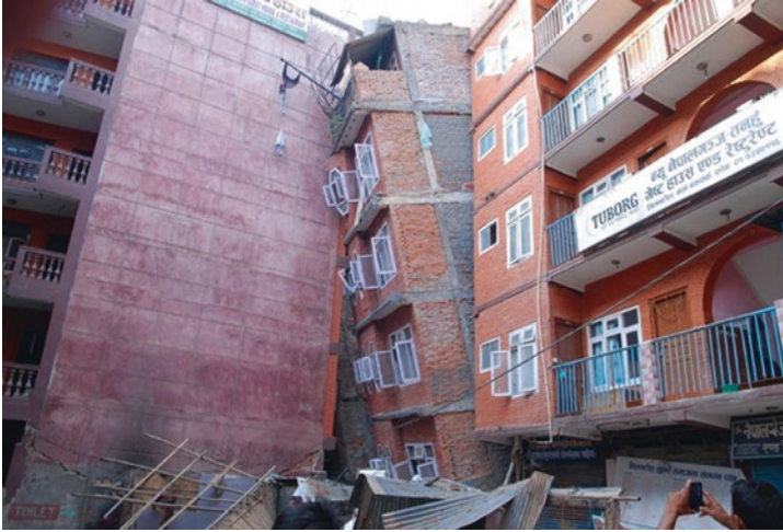
Fig. 3.1 An example of the devastation in Kathmandu (Source: NSET)
