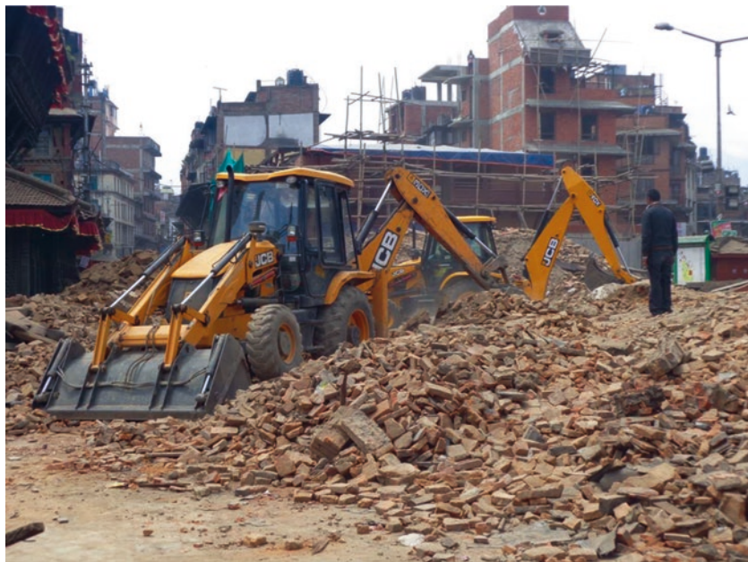
Fig. 10.1 Clearance of debris from the Kathmandu in the post-earthquake emergency phase
