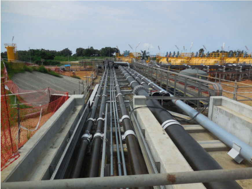
Fig. 6 Composite pipes for water transportation (Courtesy of SBPI)
