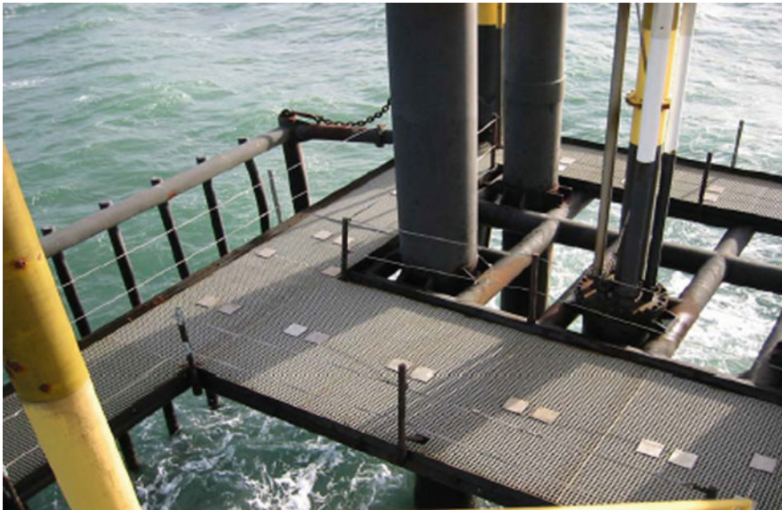
Fig. 15 Composite grating in the splash zone area of an offshore structure
