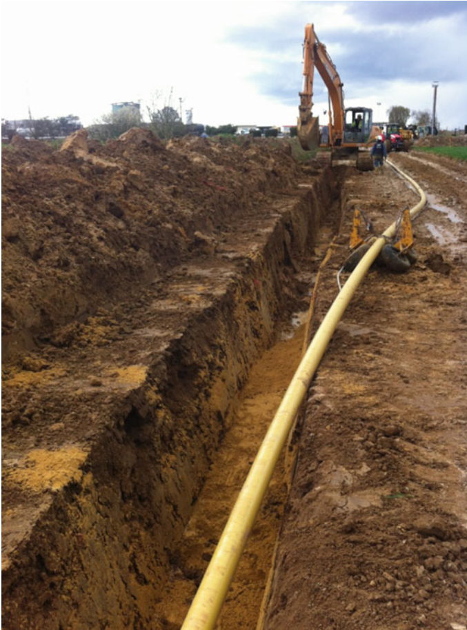
Fig. 5 Composite pipe installation for flowlines (Courtesy of SBPI)
