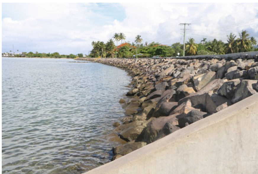
Fig. 16.6 Vaiala seawall was re-constructed in 2015, replacing the old Vaiala seawall (see Fig. 16.5). Photo credit Motisha Aiono-Solo
