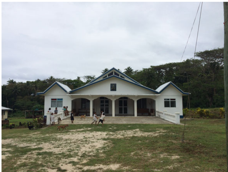
Fig. 16.3 Relocated church in southern Upolu island following the 2009 tsunami. Photo credit Miguel Esteban, 2015
