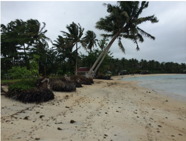
Fig. 16.7 Coastal erosion and vegetation damages due to ocean swells. Photo credit Richard Crichton, 2014
