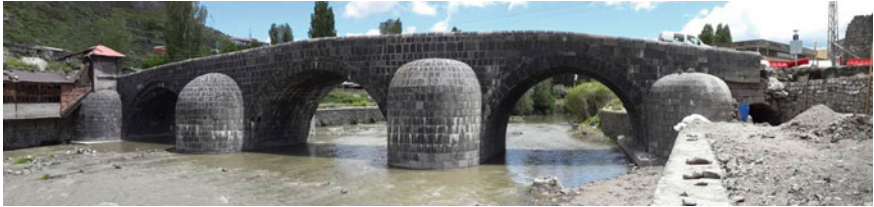
Fig. 7. The Bridge during 2013 restoration applications
