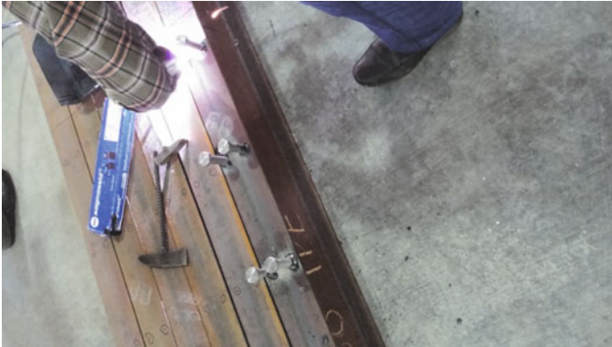
Fig. 3. Headed studs
