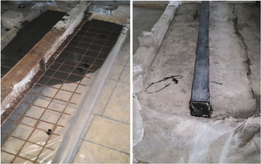
Fig. 5. Mold, concrete casting and CFRP strengthened steel concrete composite beam
