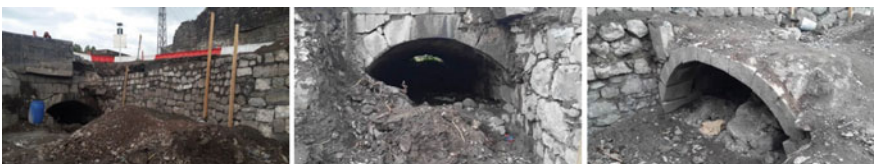
Fig. 9. Removal of the complete belt under the soil [5]
