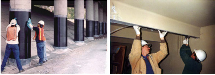
Fig. 1. FRP strengthening [5]
