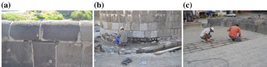
Fig. 10. a Bridge stone railings, b Bridge stones replacement, c Stone floor [5]
