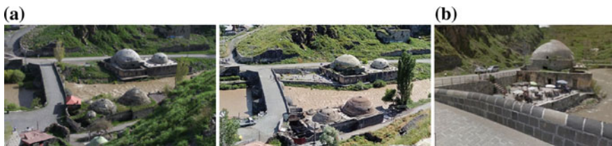
Fig. 14. Before restoration of bridge—after restoration of bridge 2013 b available sitting units
