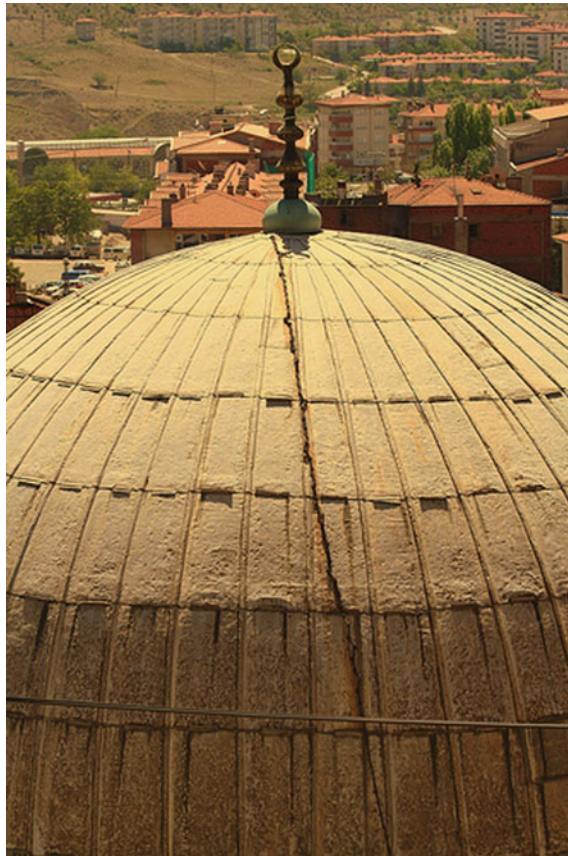
Fig. 5. Dome crack [2]
