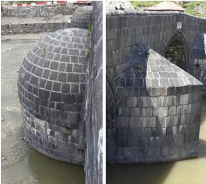
Fig. 6. Dikes and flood splitter of bridge
