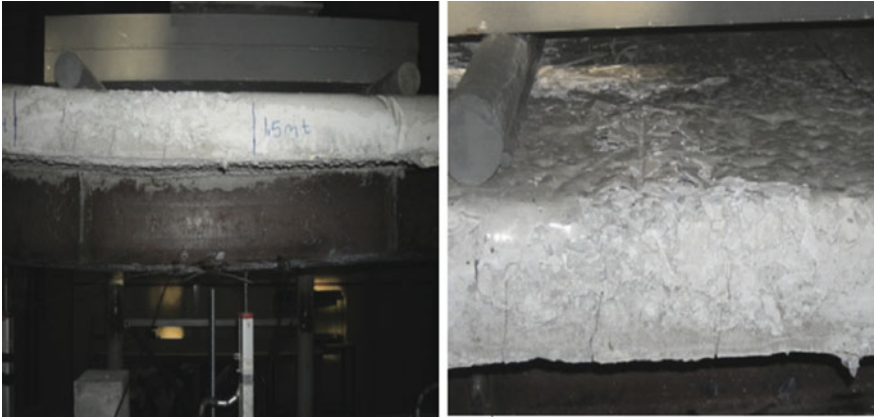
Fig. 13. Shear cracks near the loading point
