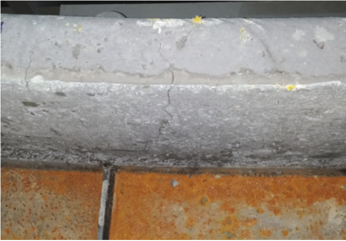
Fig. 11. Shear cracks near the loading point of un-strengthened sample
