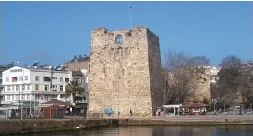
Fig. 6. Southern walls and bastion of the Sinop Castle in 2014 (from Çetin Tek archive)
