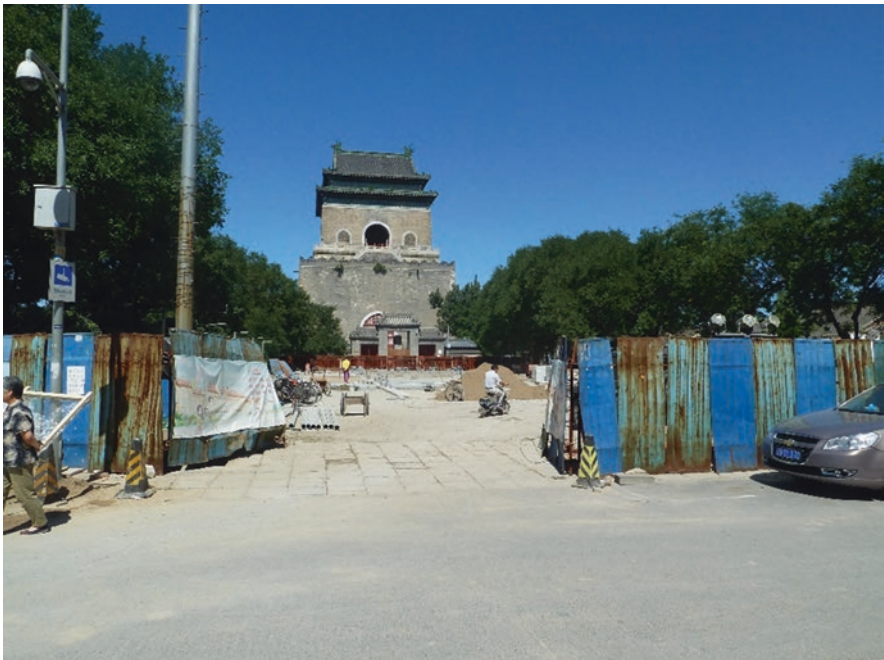
Fig. 15.4 The Drum tower during the renovation project, September 2014. © F. Graezer Bideau
