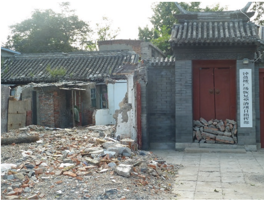
Fig. 15.3 Demolition of the Bell and Drum towers square, September 2014. © F. Graezer Bideau
