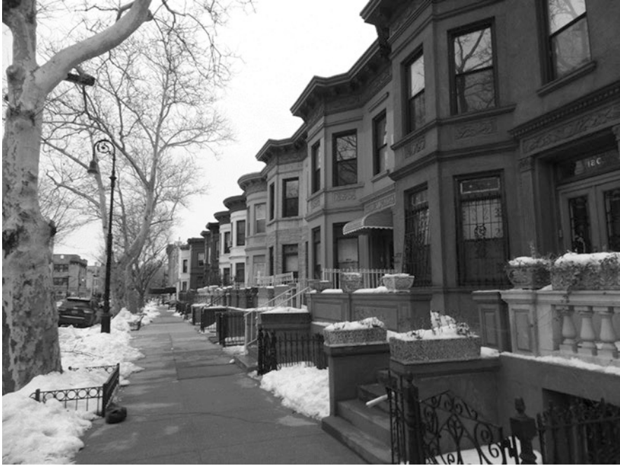
Fig. 5.2 Prospect Lefferts Gardens Sterling Street Streetscape. March 2015. Photo by Jerome Krase
