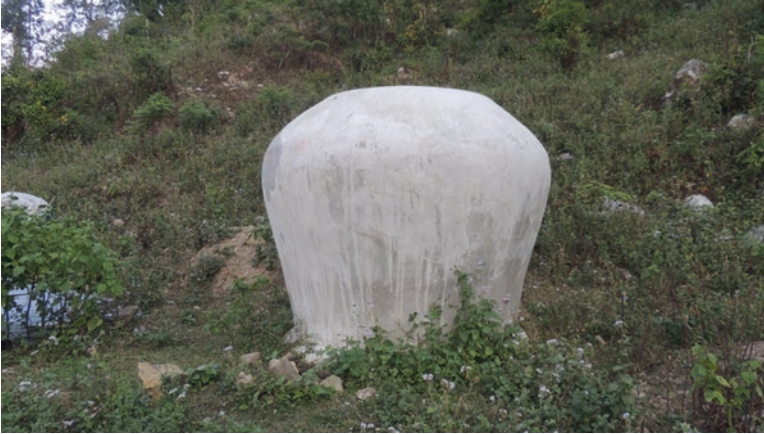
Photo 8.1 Thai jar storing water for the MUS system in the case study site, Kailali District
