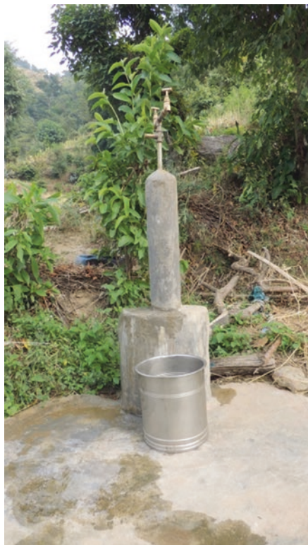
Photo 8.2 A common standing tap shared by a few households in the case study site, Doti District
