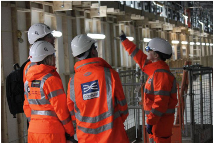
Fig. 2 The In-Site application used at crossrail’s liverpool street station site
