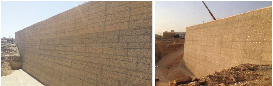
Fig. 14. Finished wall, projection-1
