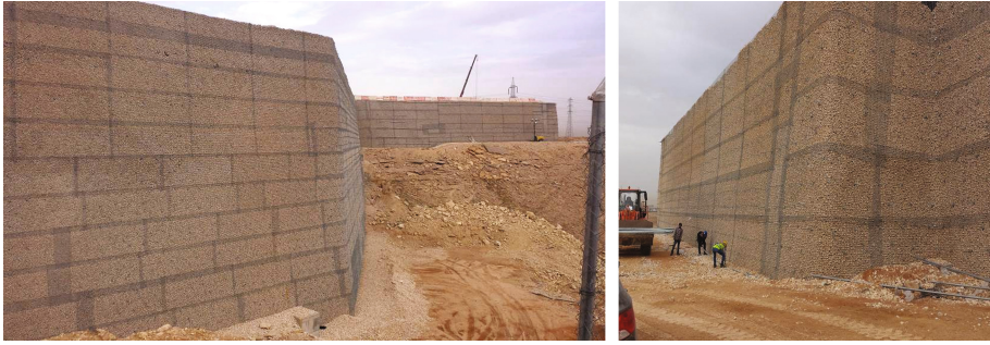
Fig. 15. Finished wall with curves and corners
