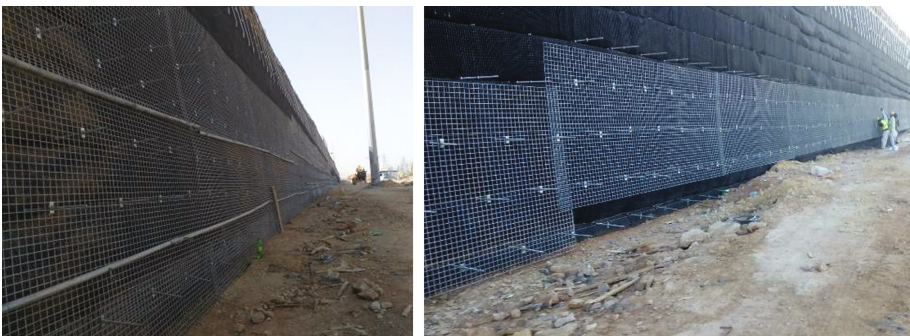
Fig. 12. Installation of Muralex steel mesh
