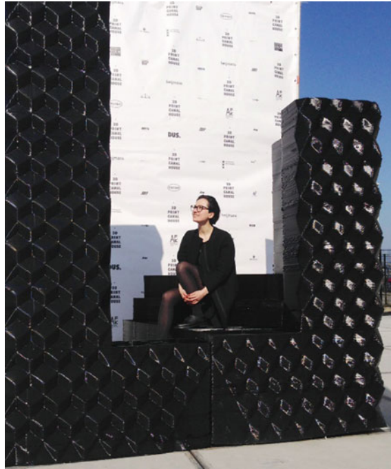
Fig. 10. 3D printed building block [42]
