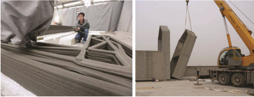
Fig. 6. 3D printed house from waste concrete [34, 35]
