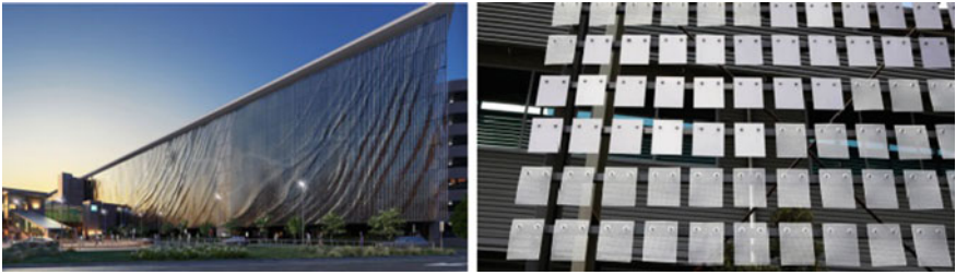
Fig. 6. Brisbane airport kinetic parking garage facade by ned kahn + UAP [20]
