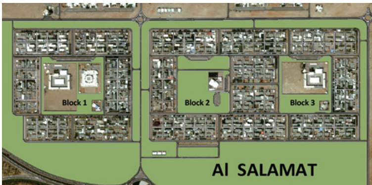
Fig. 1. Neighborhood centers distributed within the inner space of the residential blocks clusters
