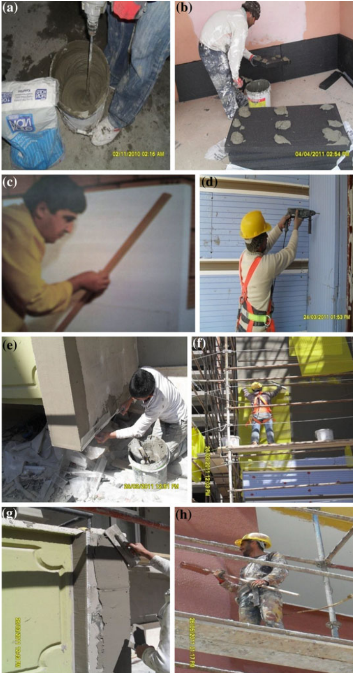
Fig. 1. The application of the coating process
