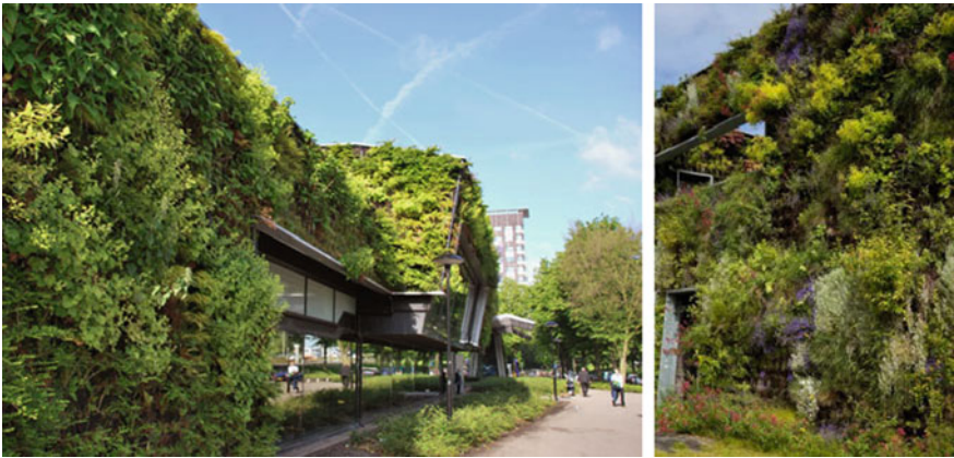
Fig. 13. The concept of vertical gardens at Sportplaza Mercator. As every wall has its own climate, over 50 different kinds of shrubs, bushes and trees have been planted in the roofs and facades of this sports centre [31]
