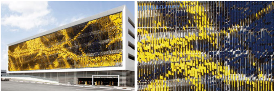
Fig. 7. Urbana studio designed an interactive aluminum facade for an existing parking structure at Eskenazi Hospital in Indianapolis. (Serge Hoeltschi) [22]
