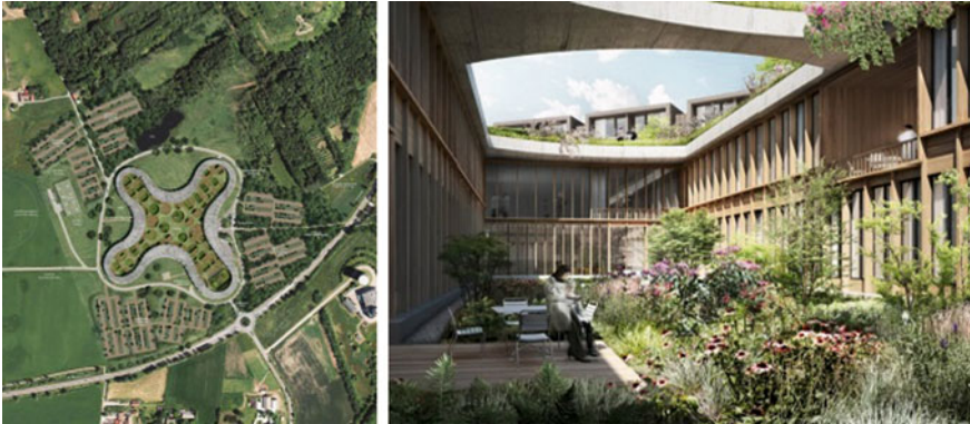
Fig. 4. New North Zealand Hospital, Hillerød, Denmark, Arch.: Herzog & de Meuron, Vilhelm Lauritzen (Competition 2013–2014, project 2014) [17]
