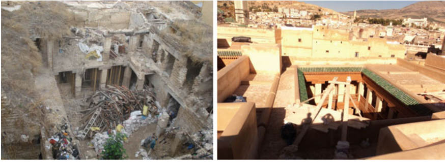
Fig. 7. Before and after restoration and rehabilitation of some buildings
