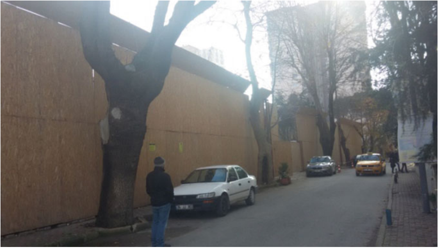
Fig. 13. An example of ongoing construction in the neighborhood
