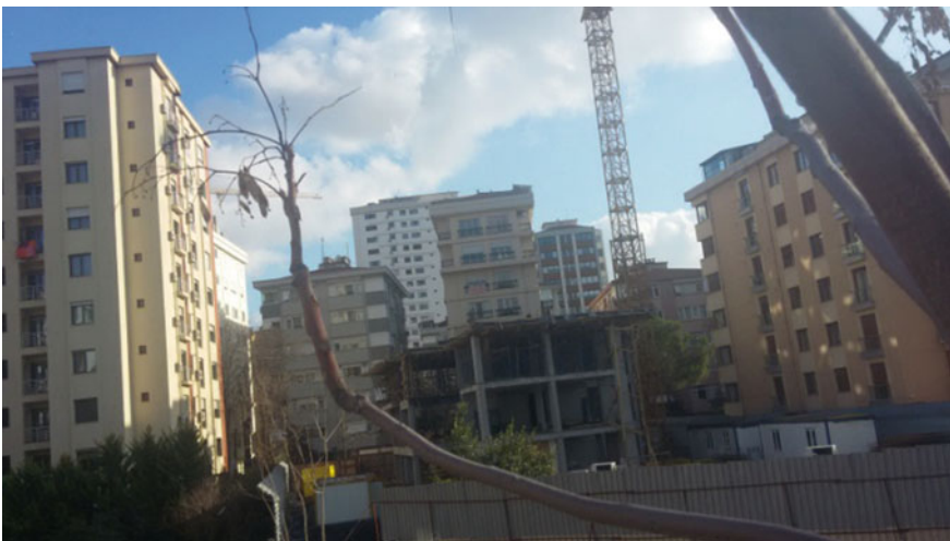
Fig. 12. An example of ongoing construction in the neighborhood
