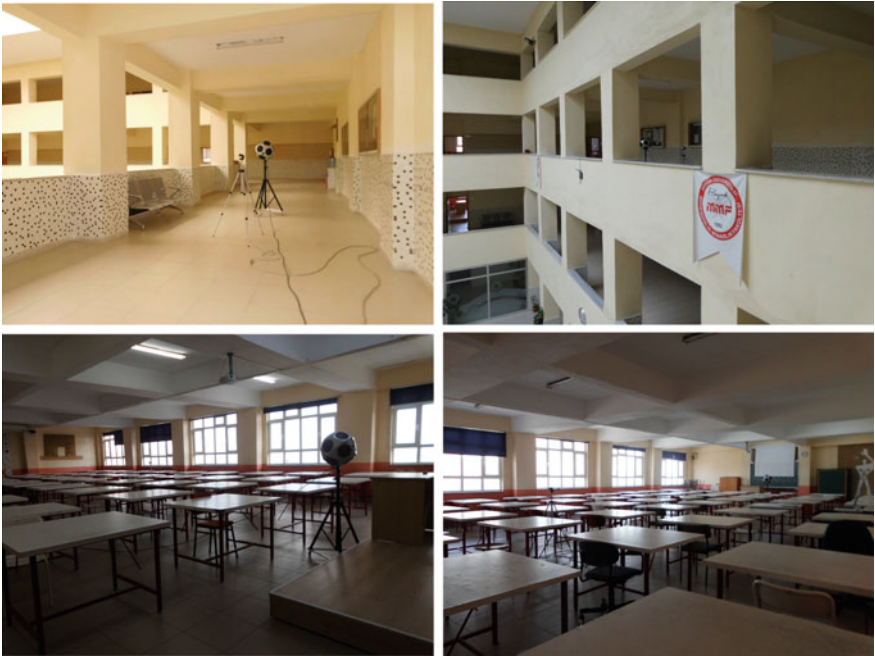
Fig. 5. Photos from the measurements at wall between the design studio-corridor
