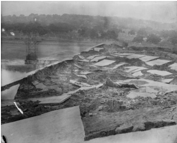
Fig. 1. Sheffield Dams failure [7]
