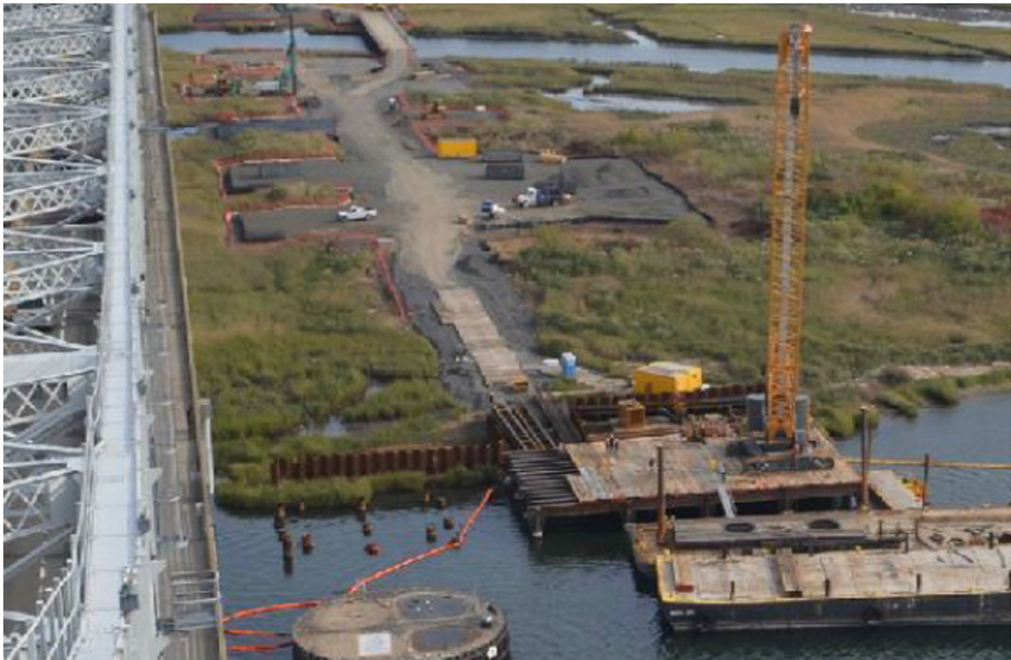
Fig. 3. Aerial photo of the proposed geogrid-reinforced-earth pile-supported embankment after construction
