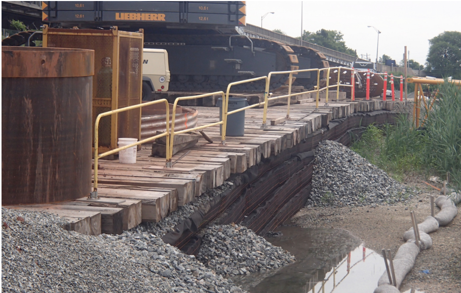
Fig. 9. Geogrid-reinforced pile-supported embankment during operation
