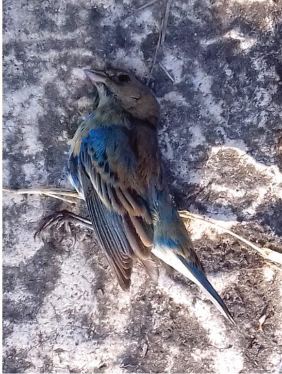
Fig. 7.2 Fatal collision of a Nearctic-Neotropical migrant passerine (Indigo Bunting – Passerina cyanea ) on a three-story building located within the city of Xalapa with important reflecting pane surface (Photo: Miguel A. Gómez-Martínez)
