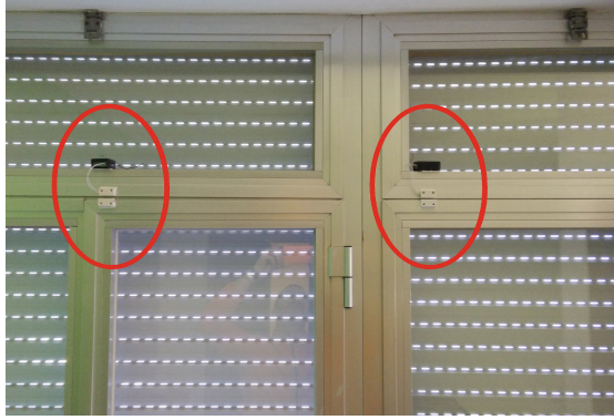
Fig. 1. Magnetic sensors for windows opening detection.
