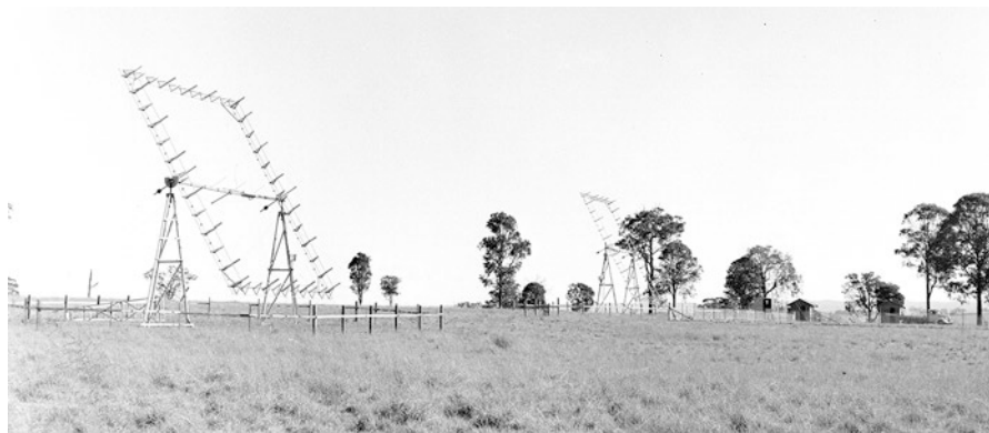
Fig. 19.53 A vista showing two of the three 101 MHz broadside antennas at Badgerys Creek (Courtesy CSIRO RAIA B2774-52)
