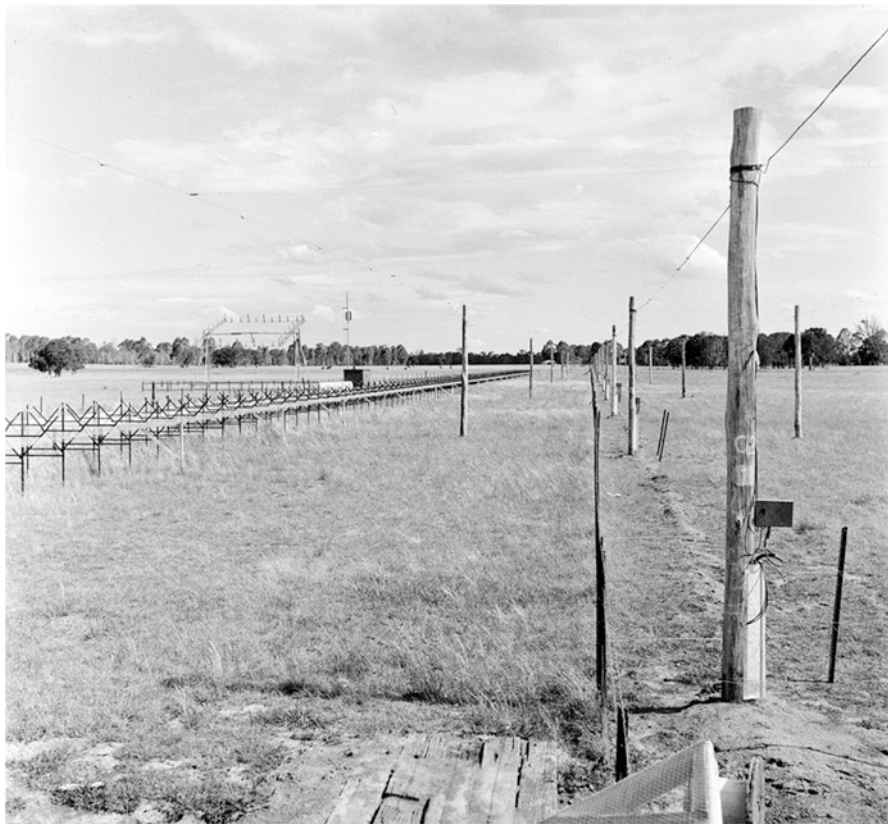
Fig. 19.79 Looking south along the N-S arm of the Shain Cross; on the left is the N-S arm of the Mills Cross, and the broadside antenna used by Alan Carter for his long baseline study of source sizes ( Courtesy CSIRO RAI AF B3868-19 )
