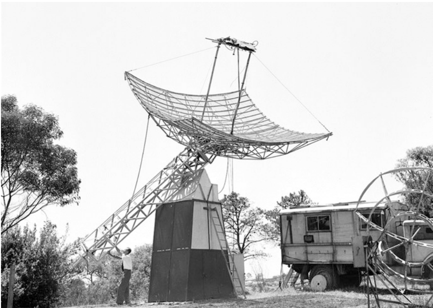
Fig. 19.32 The relocated and remounted Georges Heights ex-WWII experimental radar antenna, set up at Potts Hill for radio astronomy ( Courtesy CSIRO RAIA B2649-3)
