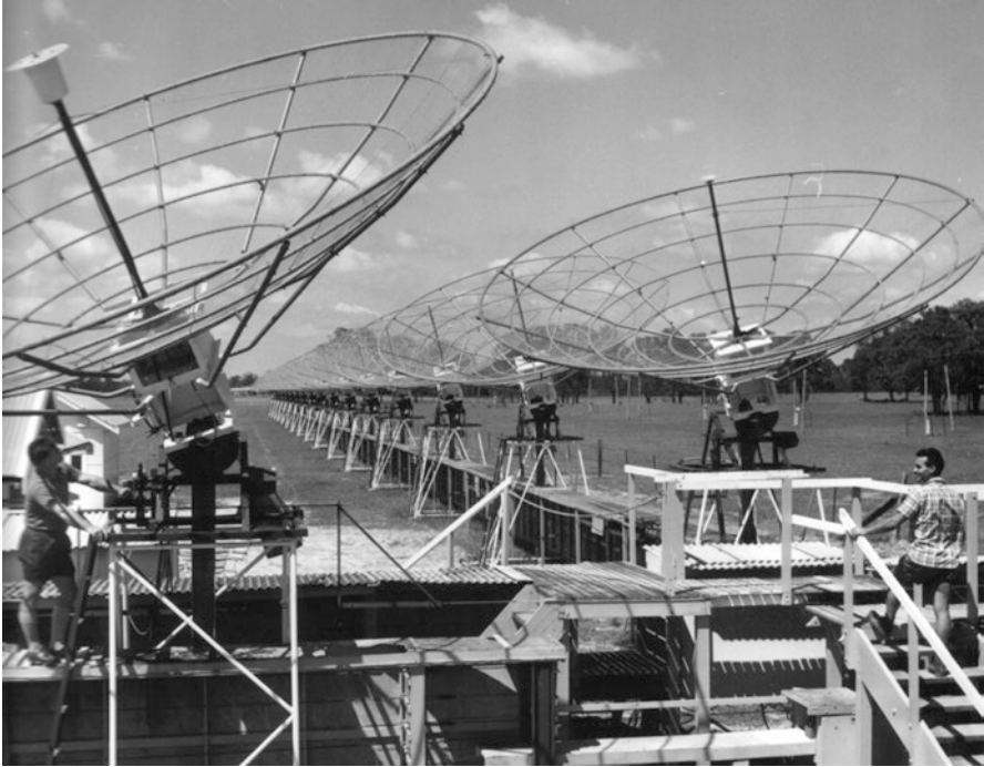
Fig. 19.83 A view looking south down the N-S arm, from near the centre of the Cross; note the superstructure erected to protect the feeder lines from the elements ( Courtesy CSIRO RAI A 9097-12 )
