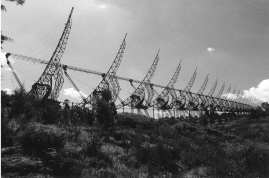
Fig. 27.17 The Ooty Radio Telescope, consisting of the 530-m long and 30-m wide cylindrical parabolic antenna placed along a north-south sloping hillside at an angle of 11.35^\circ so that its axis of rotation was parallel to that of the Earth ( Courtesy TIFR Archives)
