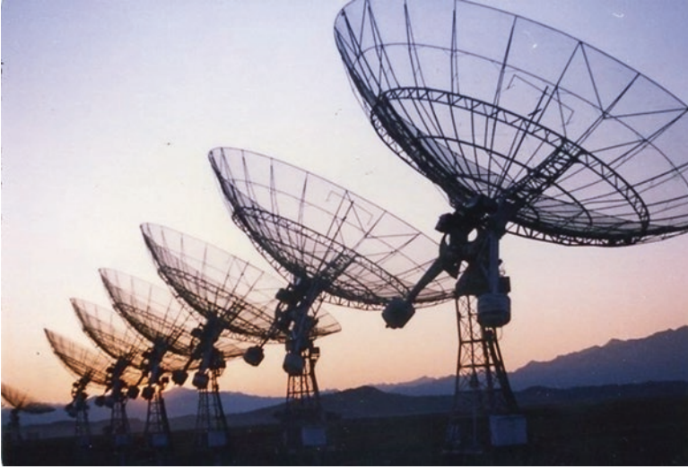
Fig. 9.4 The Miyun 28-antenna Meter Wave Aperture Synthesis Array (Courtesy Beijing Astronomical Observatory)
