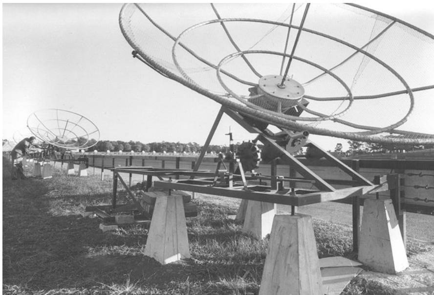
Fig. 19.40 The second 1420 MHz solar grating array, looking south; the antennas of the first solar array are only just visible in the background as a series of small white ‘dots’ (Courtesy CSIRO RAIA 3116-1)
