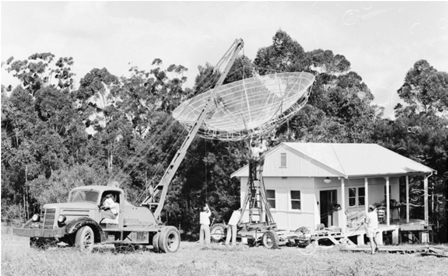
Fig. 19.90 The Murraybank field station, showing installation of the 6.4-m dish, and the adjacent building which housed the H-line receiver ( Courtesy CSIRO RAIA B3973-4)
