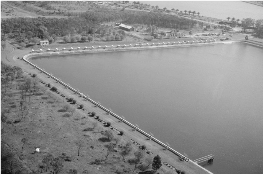
Fig. 27.6 A view looking south-west across the two Potts Hill water reservoirs in 1953, showing Christiansen’s solar grating arrays along the banks of the eastern reservoir. The E–W array consisted of 32 elements and the nearer N–S array just 16 elements ( Courtesy CSIRO RAIA: 3475-1 )
