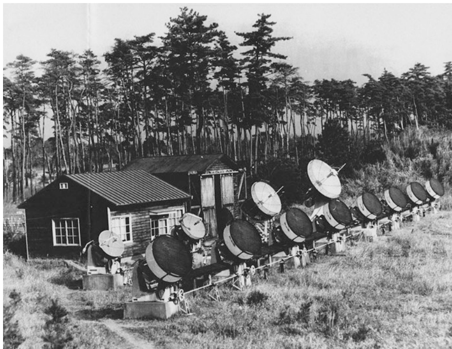
Fig. 6.11 The expanded 8-element solar grating array, complete with polarisation screens, and behind it the four total power radiometers that monitored the Sun at 1000, 2000, 3750 and 9400 MHz ( Courtesy Tanaka Family )
