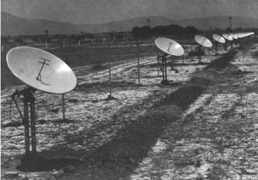
Fig. 27.16 A view of the east-west grating array consisting of twenty-four 6-ft diameter dishes built at Kalyan, near Mumbai, in 1965 ( Courtesy TIFR Archives )
