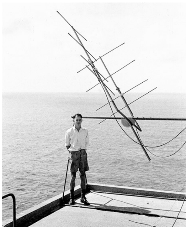
Fig. 19.6 A May 1947 close-up of John Bolton and the 100 MHz twin Yagis mounted on the roof of the cliff-side WWII block-house at Dover Heights (Courtesy CSIRO RAIA B1031-7)
