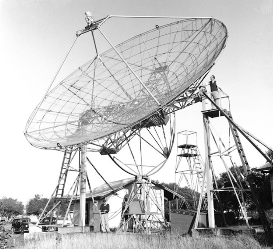
Fig. 19.45 The 11-m parabola constructed for H-line work in 1952–1953, with the receiver hut in the background ( Courtesy CSIRO RAIA 3679-1 )
