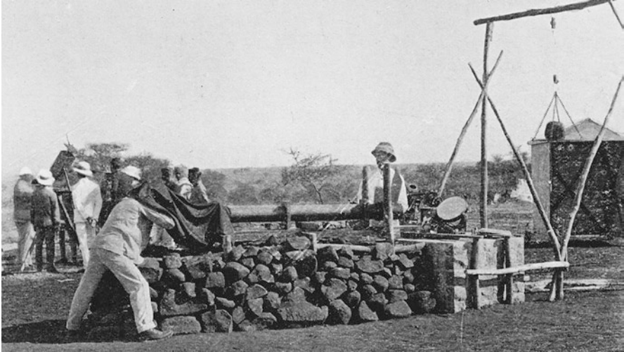
Fig. 26.14 Professor Naegamvala's horizontal photographic telescope at Jeur in 1898 (after Maunder 1899: 81)
