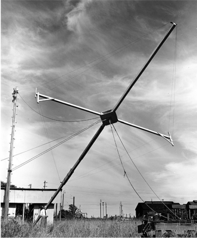
Fig. 19.58 The 70–130 MHz rhombic aerial at the short-lived Penrith field station ( Courtesy CSIRO RAIA B2086-1 )
