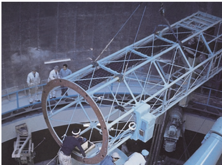
Fig. 5.1 Installation of the Okayama 1.88-m Reflector ( Courtesy NAOJ )
