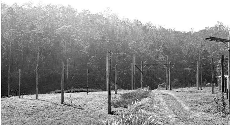
Fig. 19.27 A photograph showing part of the second 18.3 MHz array at Hornsby Valley ( Courtesy CSIRO RAIA B2802-5 )
