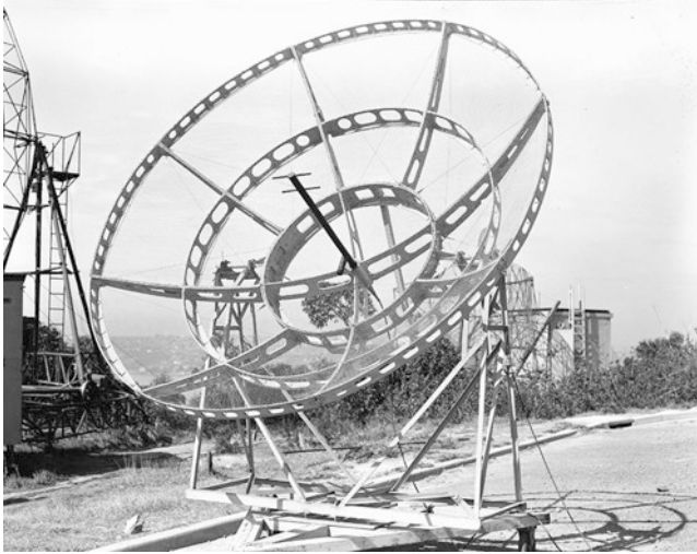
Fig. 19.21 One of the portable 3.05-m dishes set up at Georges Heights ( Courtesy: CSIRO RAI A 1511 )
