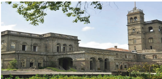
Fig. 24.34 A photograph of part of the Government College of Science in Poona ( http://educrrib.com/college/4310/college-of-engineering-coep-pune )
