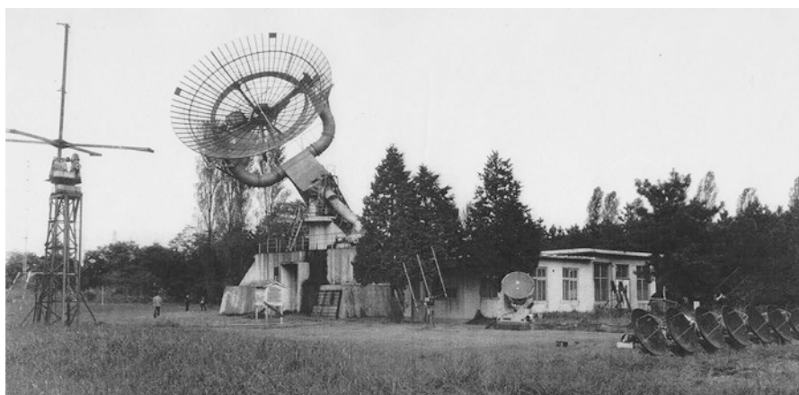
Fig. 6.7 Left of centre is the 10-m equatorially mounted dish erected at the TAO in 1953, which was used to monitor solar radio emission at 200 and 3000 MHz; on the left is the rhombic aerial of one of the solar radio spectrographs, and on the far right is a grating interferometer that was subsequently installed to identify the positions of active regions at 9000 MHz ( Courtesy National Astronomical Observatory of Japan )
