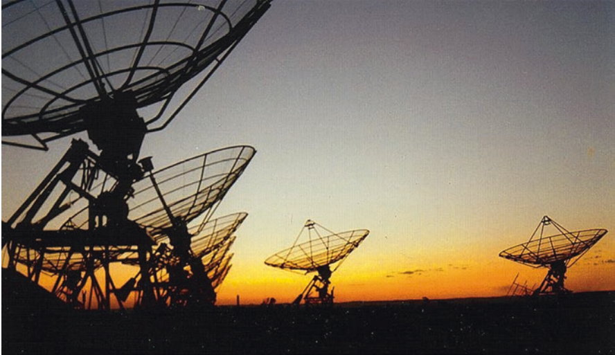
Fig. 9.2 View of the central part of the Chris Cross, looking west at sunset. This array comprised E-W and N-S arms each with 32 steerable parabolic antennas of 5.8-m diameter. This was the world's first crossed-grating interferometer and it was used to produce daily isophote maps of solar emission at 1423 MHz ( Courtesy John Leahy )
