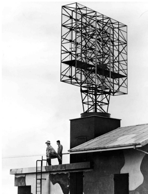
Fig. 18.5 The 200 MHz wartime radar antenna for shore defense, consisted of a 36-dipole array rotatable only in azimuth, at Dover Heights (1941). This and a similar antenna at Collaroy were used by Pawsey's group in 1945–1946 as sea-cliff interferometers for observations of the rising Sun (Courtesy ATNF RAIA B81-16)
