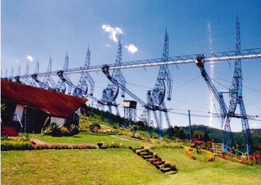
Fig. 27.18 Another view of the Ooty Radio Telescope; reflections of sunlight by 1100 stainless steel wires are seen on the right (Courtesy TIFR Archives)
