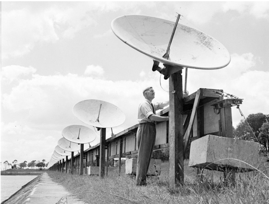
Fig. 19.37 Chris Christiansen and the first 1420 MHz solar grating array at Potts Hill, looking east (Courtesy CSIRO RAIA 2976-1)
