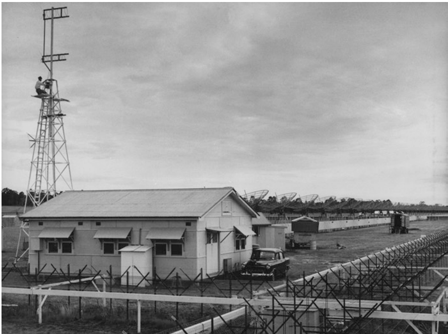
Fig. 19.73 A close-up of the centre of the Mills Cross, showing individual dipoles, and the receiver hut and microwave link used for long baseline interferometry; in the background are some of the dishes of the Chris Cross ( Courtesy CSIRO RAIA B5689-8 )
