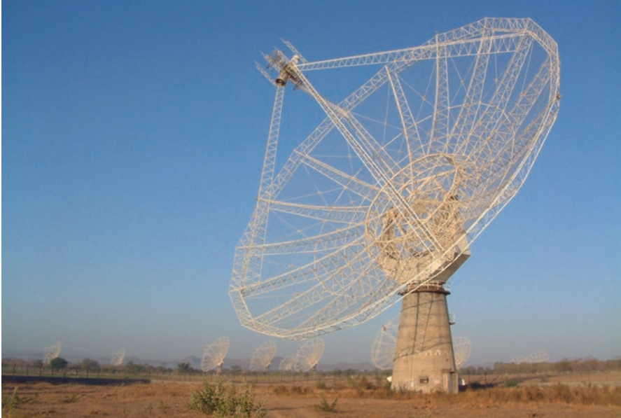
Fig. 27.19 A close-up view of one of the thirty 45-m diameter fully steerable parabolic dishes of the Giant Metre Wavelength Telescope located at Khodad, near Pune, in western India. A few dishes of the central array of the GMRT are also visible in this photograph ( Courtesy Prem Kumar, NCRA-TIFR Archives)
