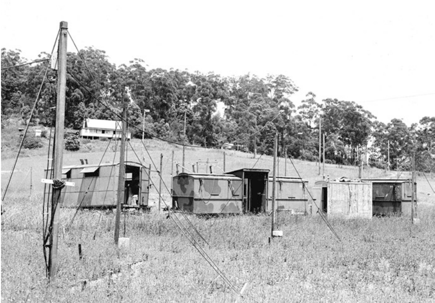
Fig. 19.23 The assemblage of huts, trailers, poles and wiring associated with the Moon-bounce experiments (Courtesy CSIRO RAIA 1266-5)
