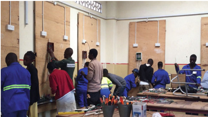
Fig. 1 YCTC students during a practical lesson of electric wiring
