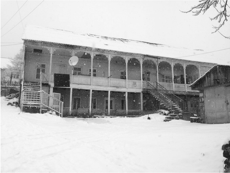
Fig. 5 A traditional building in the village of Sanahin
