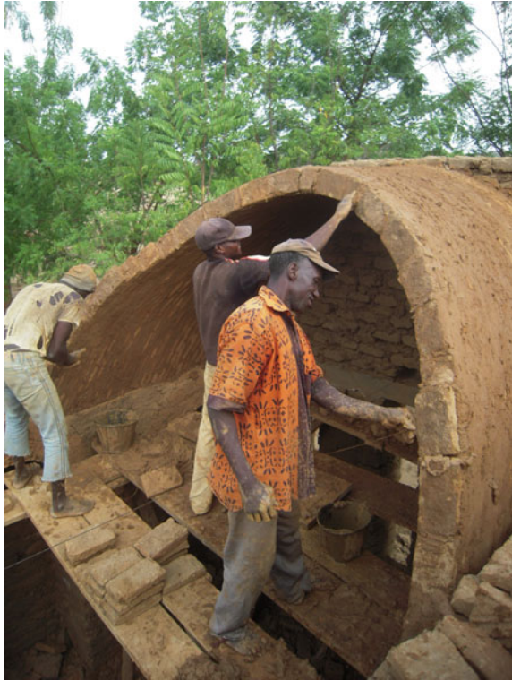
Fig. 4 Nubian Vault construction site. Photo credits: All pictures are made by caravatti_caravatti architetti
