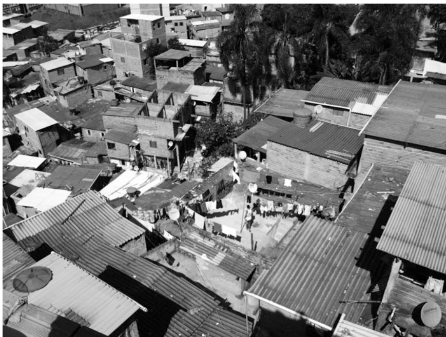
Fig. 1 The roofs of Paraisópolis (Photo of the author)
