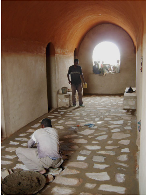
Fig. 5 Bolmò_Republic of Mali Nubian Vault interior. Photo credits: All pictures are made by caravatti_caravatti architetti
