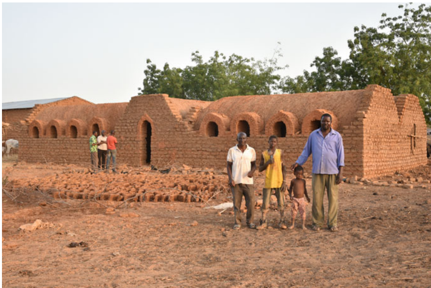
Fig. 1 N'golofalà_Republic of Mali Nubian Vault private house. Photo credits: All pictures are made by caravatti_caravatti architetti
