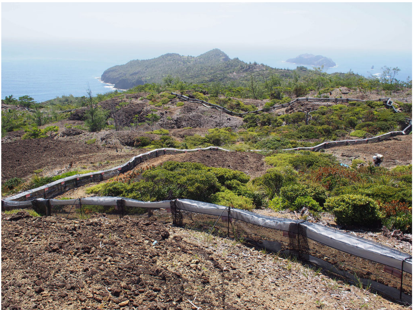
Fig. 6.8 Fence constructed in Anijima to prevent expansion of Green Anoles
