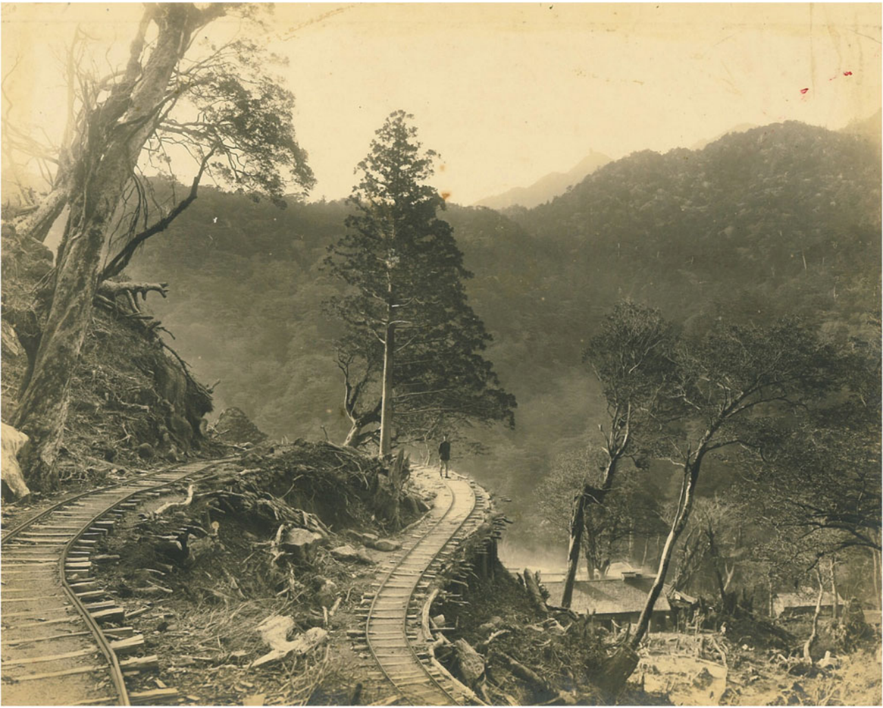
Fig. 7.3 A photo of a newly constructed timber railway in Yakushima during the 1920s. Source: Yakushima Forest Ecosystem Conservation Center
