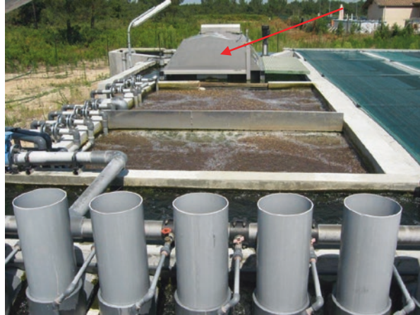
Fig. 36.2 Water treatment devices in sturgeon farm (Nurseteich Farm, France). Red arrow shows the rotative filter (mechanical filter) (Photo: Mauduit)
