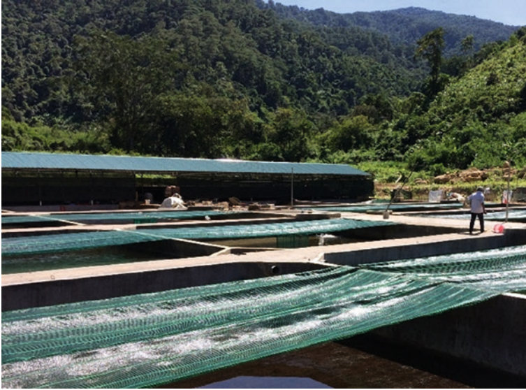
Fig. 38.11 Sub-square concrete tanks in Vietnam. Each of the four 90° angles is changed for a 45° wall to limit the accumulation of wastes and then the deterioration of water quality. Note that tanks are partially shadowed (credit V. Chipinov)
