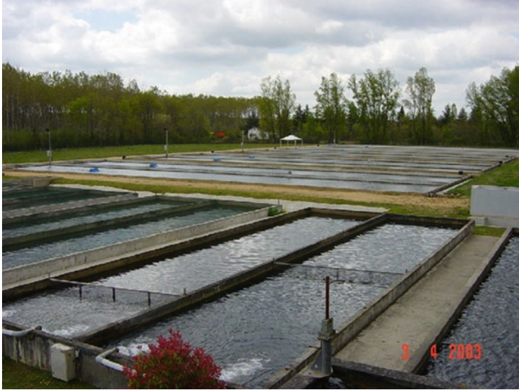
Fig. 38.8 Small twin raceways with a low-water depth separated into two parts. Prunier Manufacture sturgeon farm, South West of France (credit P. Williot)
