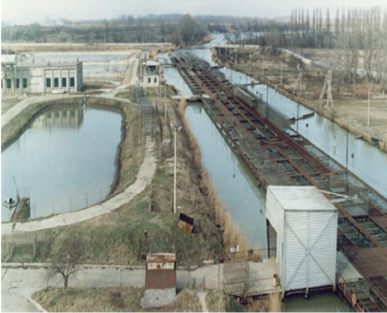
Fig. 38.12 One of the largest sturgeon cage farms in Russia, the Kuban Sturgeon Farming Institute, the Krasnodar Region. Cages are arranged by the side of the other in a canal supplied by industrial warm water (right part of the photo) (credit M. Chebanov)
