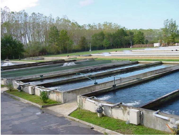
Fig. 38.5 Small twin raceways with a low-water depth. Note that some are covered by a net to avoid avian predation, and one is enriched with oxygen by an aerator. Prunier Manufacture sturgeon farm, South West of France (credit P. Williot)
