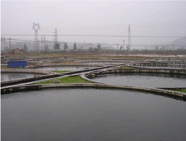
Fig. 38.10 Large concrete circular tanks for rearing Siberian sturgeon in China (credit M. Chebanov)
