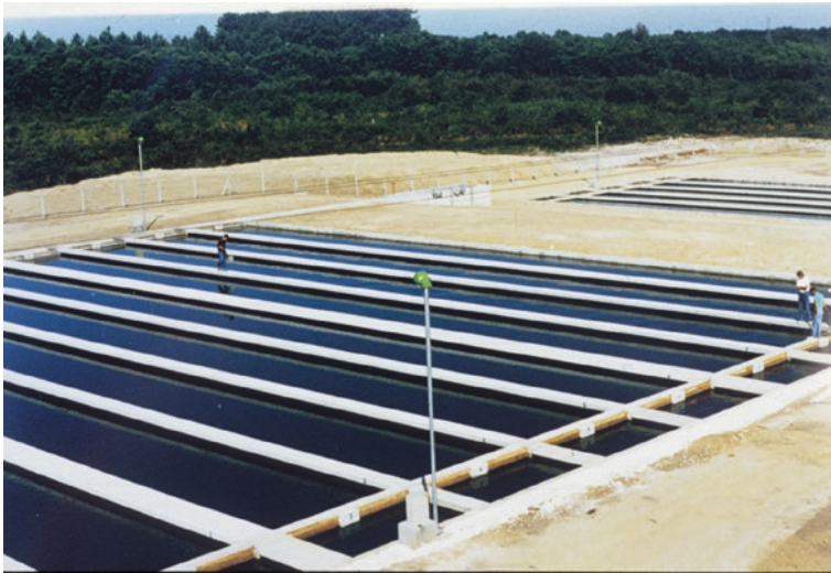
Fig. 38.2 Classical sized concrete raceways arranged in parallel. The water inlet canal is on the right down corner. Primary step of building of the sturgeon farm L' Esturgeonnaire, South West of France (credit Esturgeonnaire Co)
