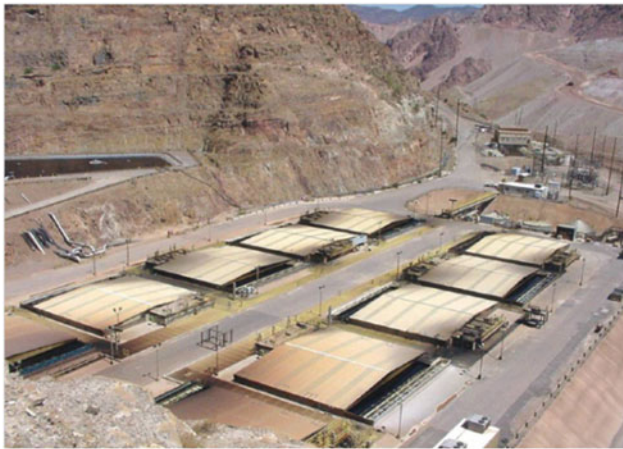
Fig. 6.9 Simplified flow sheet of the leaching and metal recovery by solvent extraction (a) electrowinning plant at Konkola Copper Mines, Zambia (Sole et al. 2005) and (b) solvent extraction plant Morenci, Arizona, USA (Marsden 2006)
