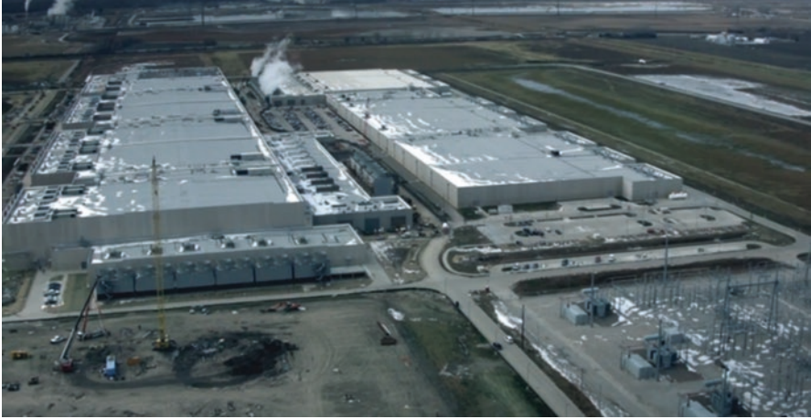
Fig. 13.1 Google's large DC facility in Council Bluffs, Iowa
