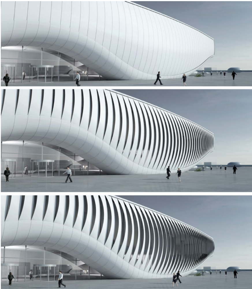
Fig. 1 Soma architecture, One Ocean: Expo 2012 Thematic Pavilion, Yeosu-kinetic media façade consisting of GFRP louvers
