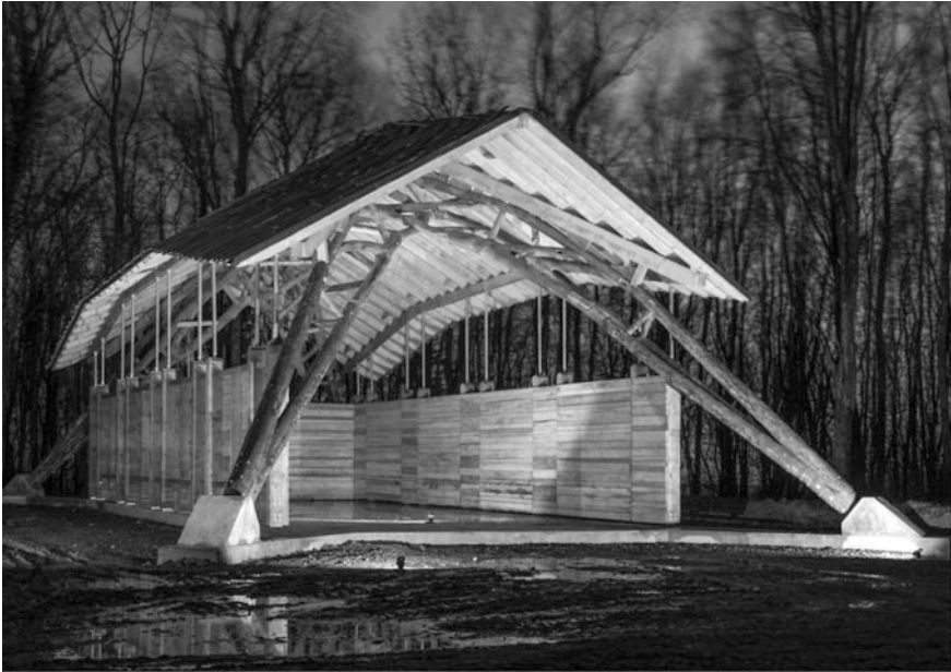
Fig. 1 AA Hooke Park. Wood chip barn
