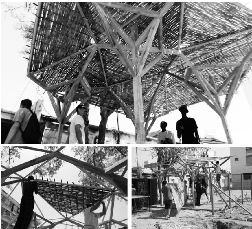
Fig. 6 Open air lab, construction process ( below )
