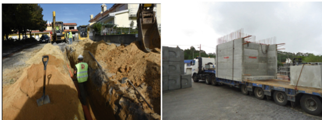
Fig. 2. Construction of drainage networks for sewage and water supply
