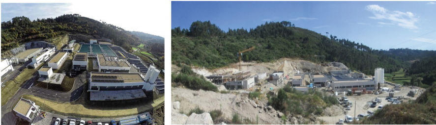
Fig. 1. Construction of large sewage treatment plant.
