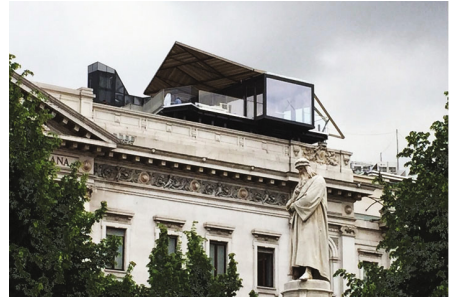
Fig. 8. Restaurant “Priceles Milano” on the top of Banca Commerciale Italiana building in Piazza della Scala during the Expo 2015, phot. A. Bonenberg
