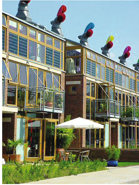
Fig. 2. Zero Energy Development (BedZED) in London's Hackbridge, technical details in designer forms, phot. A. Bonenberg
