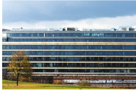
Fig. 6. Poznan, an office building from 2010 is dominated by industrial “roofscape” of the ventilation and air conditioning equipment, phot. T. Bardzinska-Bonenberg
