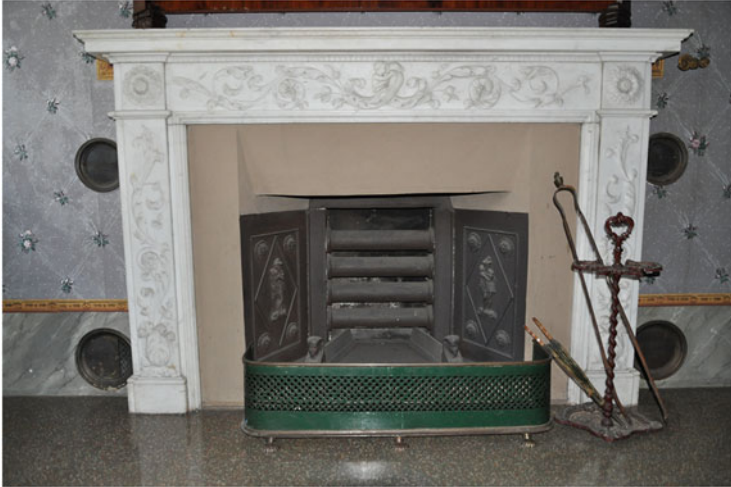
Fig. 9.3 Fireplace surrounded by four heating vents
