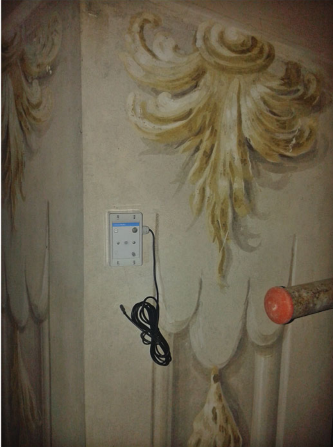
Fig. 10.5 “Node 48” at 5.65 m from the ground
