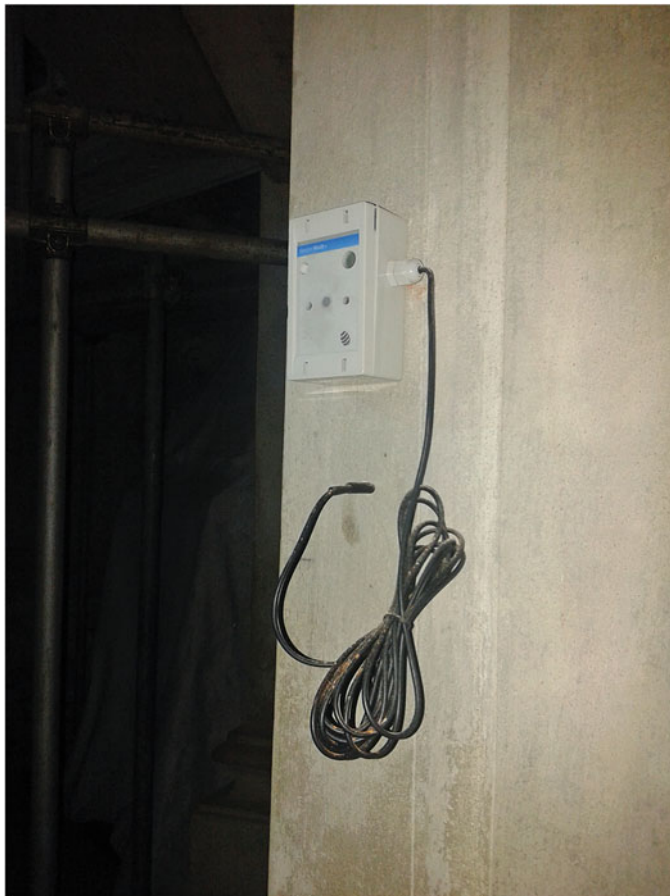
Fig. 10.4 “Node 60” at 1.65 m from the ground
