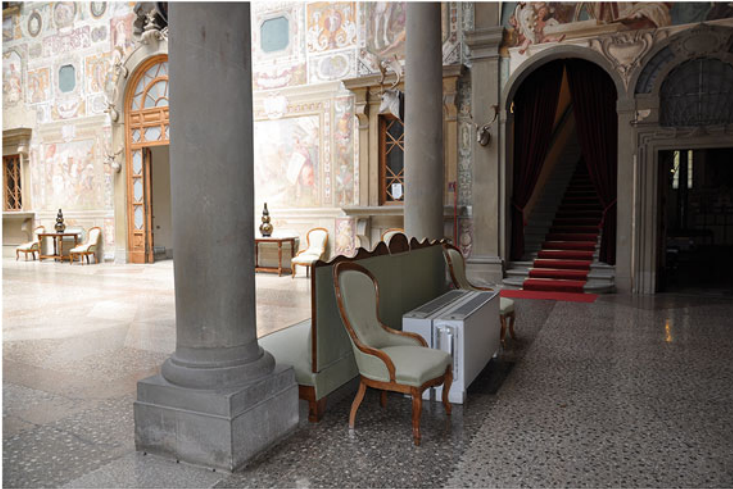
Fig. 9.5 The fan coils installed in the courtyard
