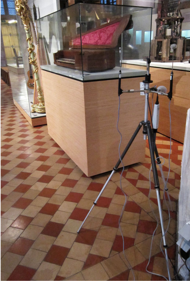
Fig. 11.5 Innova MM 0036, MM 0038, MM 0060, and Vaisala GM70 sensors during the installation on dedicated support
