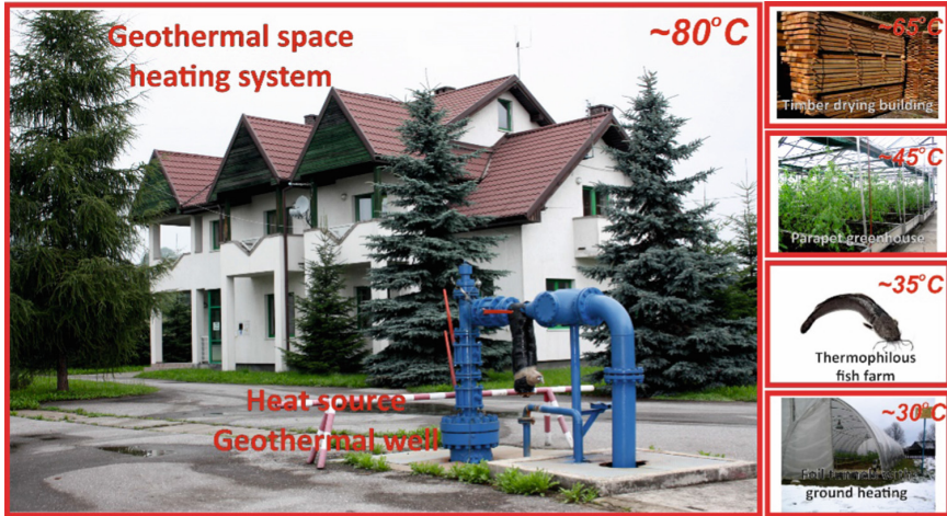
Fig. 2. The cascade system for the utilisation of geothermal energy in PAS MEERI in Poland.
