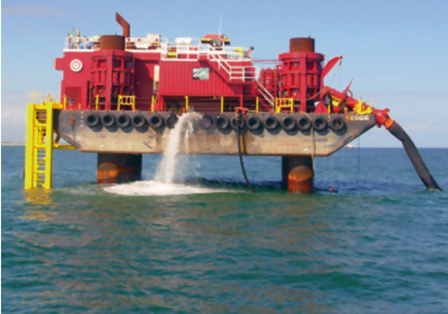
Fig. 10.5 Pipeline booster pump. Courtesy of Great Lakes Dredge & Dock
