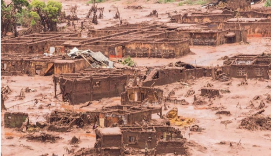
Fig. 51.3 Damage from the tailings pond failure in Brazil in 2015. Credit: Vitor Machado Lira
