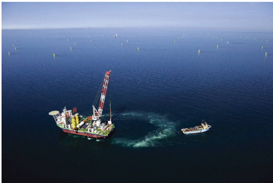
Fig. 9.2 Bubble curtain against underwater ramming noise at OWF Godewind (© DONG Energy)
