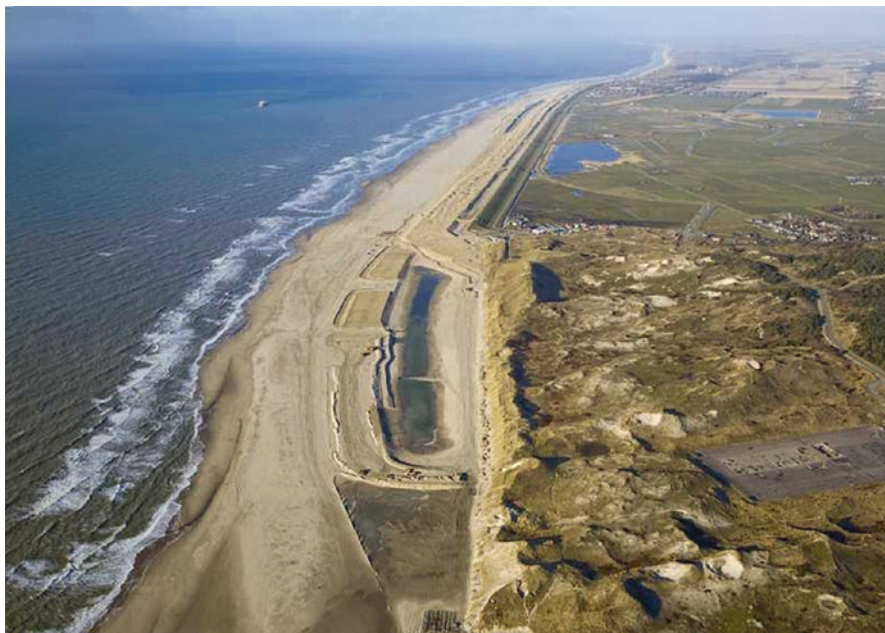
Fig. 10.16 Coastal reinforcement dredging project in the Netherlands. Courtesy Van Oord–Boskalis
