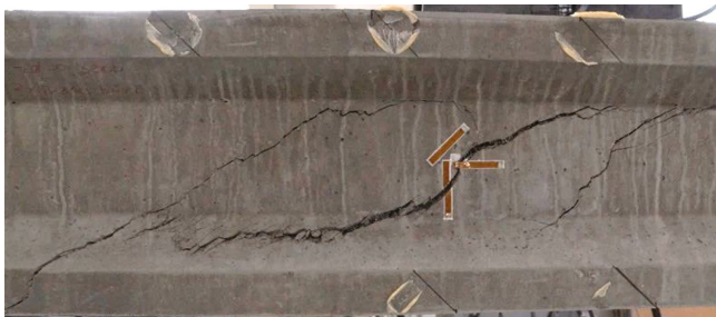
Fig. 2. Failure mode of beam B29 (no stirrups, 1 Vol.-% fibres)
