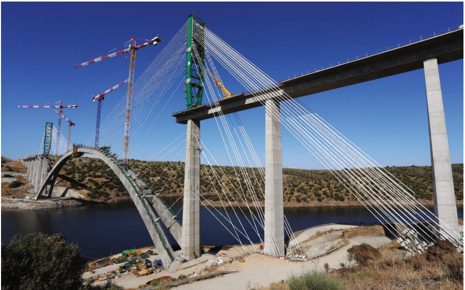
Fig. 4. Almonte Viaduct under construction.
