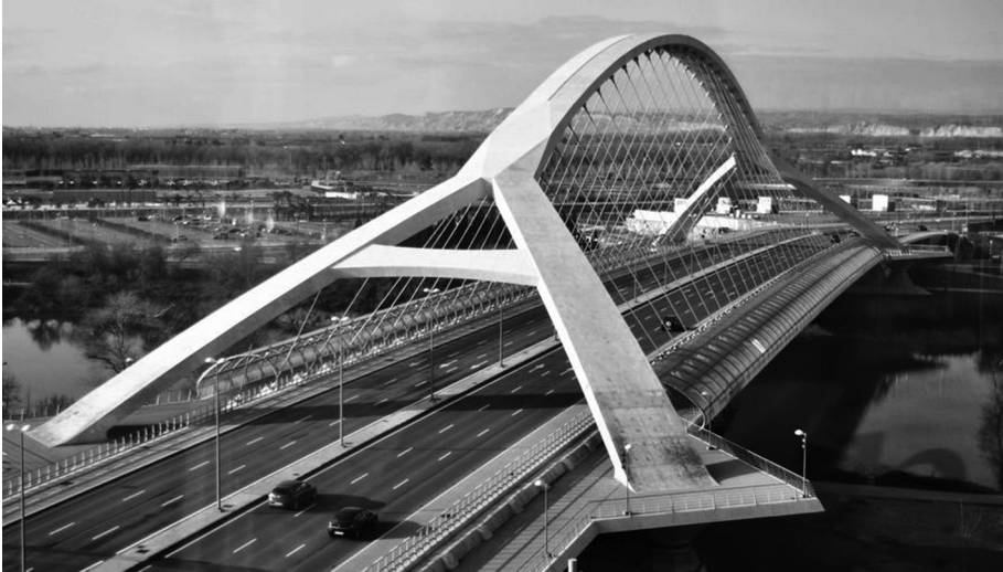
Fig. 1. Third Millennium Bridge over River Ebro.
