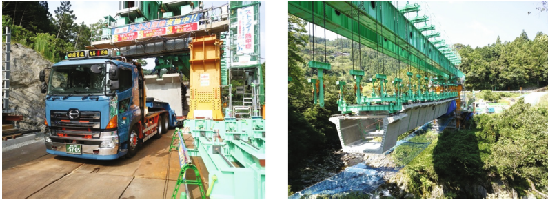
Photo 1. Erection situation at site.
