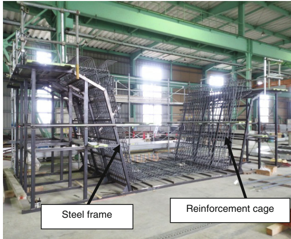
Photo 2. Prefabrication of reinforcement.
