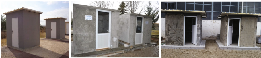
Fig. 3. Demo buildings installed in EU sites (Spain, Turkey, Romania) using SUS-CON prefabricated components and ready-mixed concretes.
