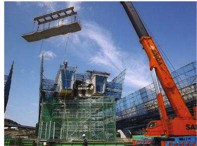
**Photo 2.** Erection of precast floor slab (Outbound lane)
