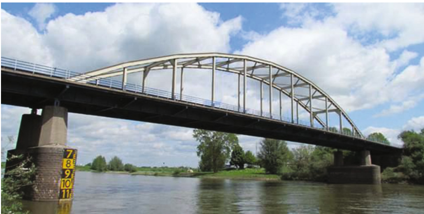
Fig. 5. Bridge across river IJssel near Doesburg (NL)
