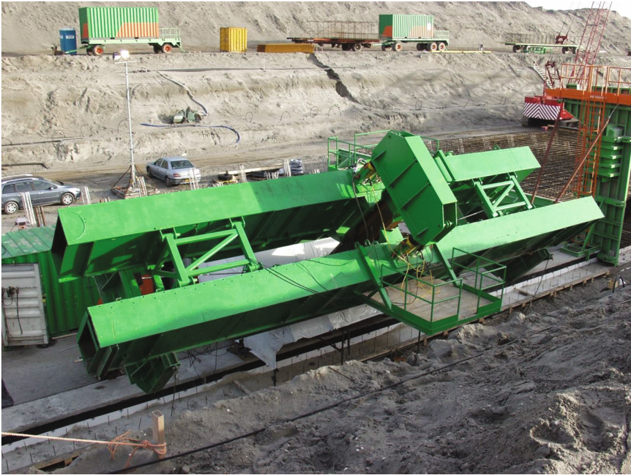
Fig. 2. Anchor pile trial load test setup
