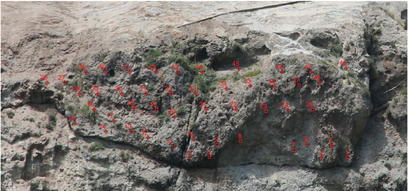
Fig. 31 Positioning of the the 48 installed dowels
