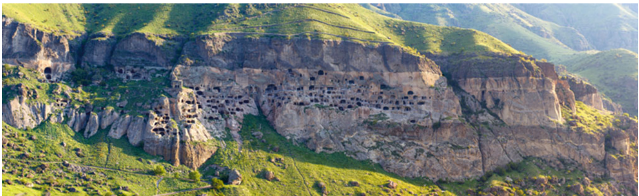
Fig. 12 General view of rock-cut city of Vardzia (Georgia)
