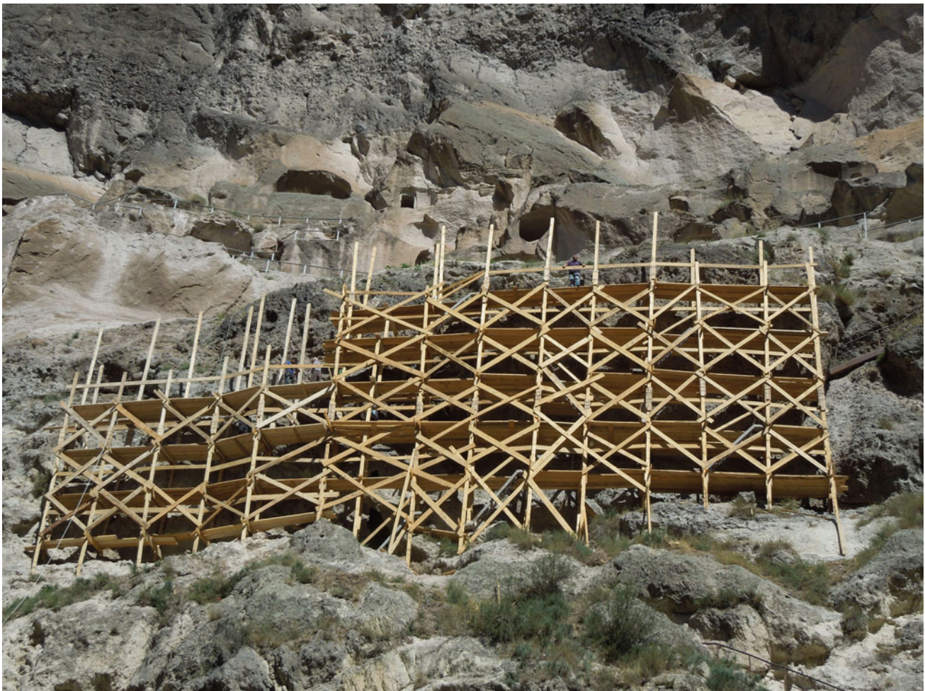
Fig. 30 The wood scaffolding realised in Vardzia
