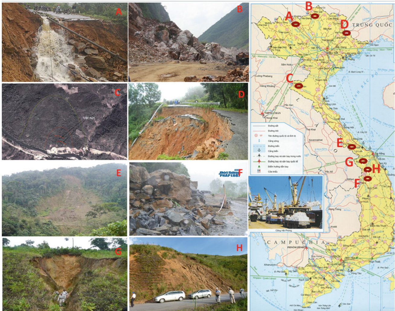
Fig. 1 Some pictures of landslides that have taken place and their location on a map of the Vietnamese transport system
