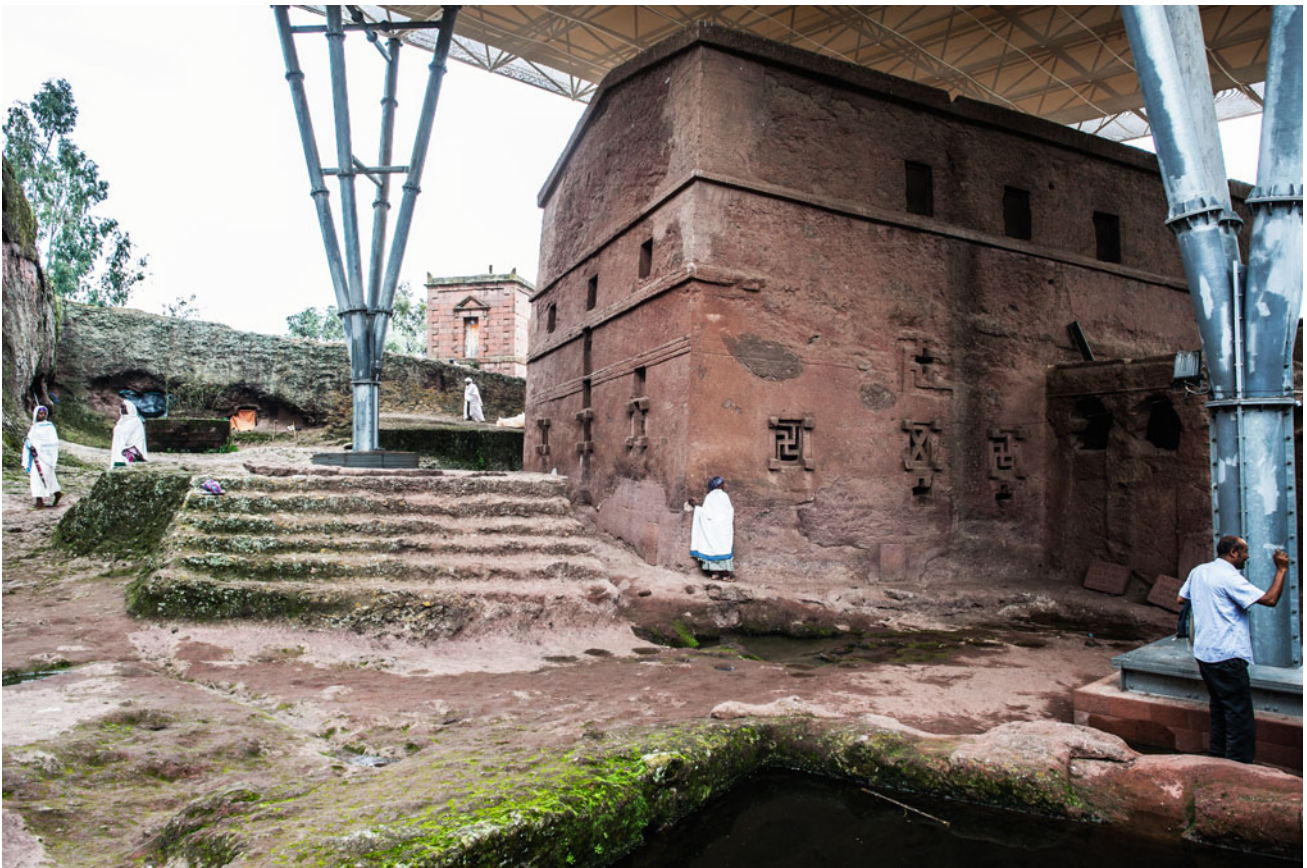
Fig. 25 The modern shelters covering the rock-hewn churches of Lalibela (Ethiopia) (source www.flickr.com )
