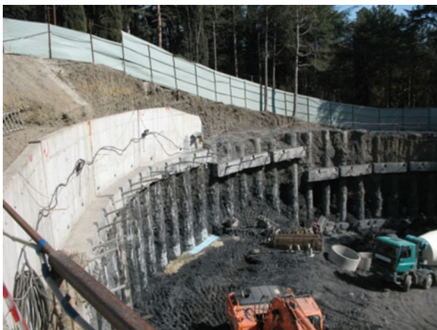
Fig. 4 Stages of construction: pit when arranging the 2nd tier of beams for anchor fixing
