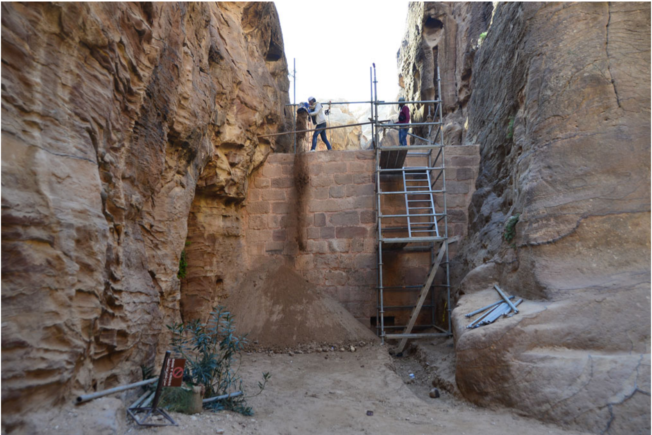
Fig. 26 Manual and proper cleaning of stone dams, to protect the Siq of Petra from flash flood
