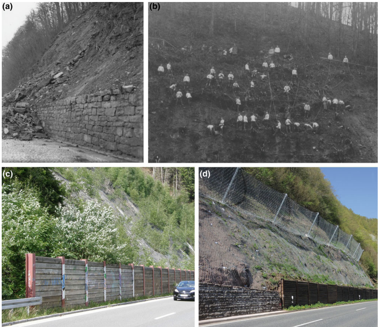
Fig. 3 Development of mitigation measures in southern Lower Saxony, NW Germany. a Rockslide event (02/1937) in the Upper Weser area. The drywall in the front stabilizes slope with no protection against rockfalls/slides. b Removal of loose rock and vegetation in the Upper Weser area in 1936. c Combination of steel buttress/wooden
