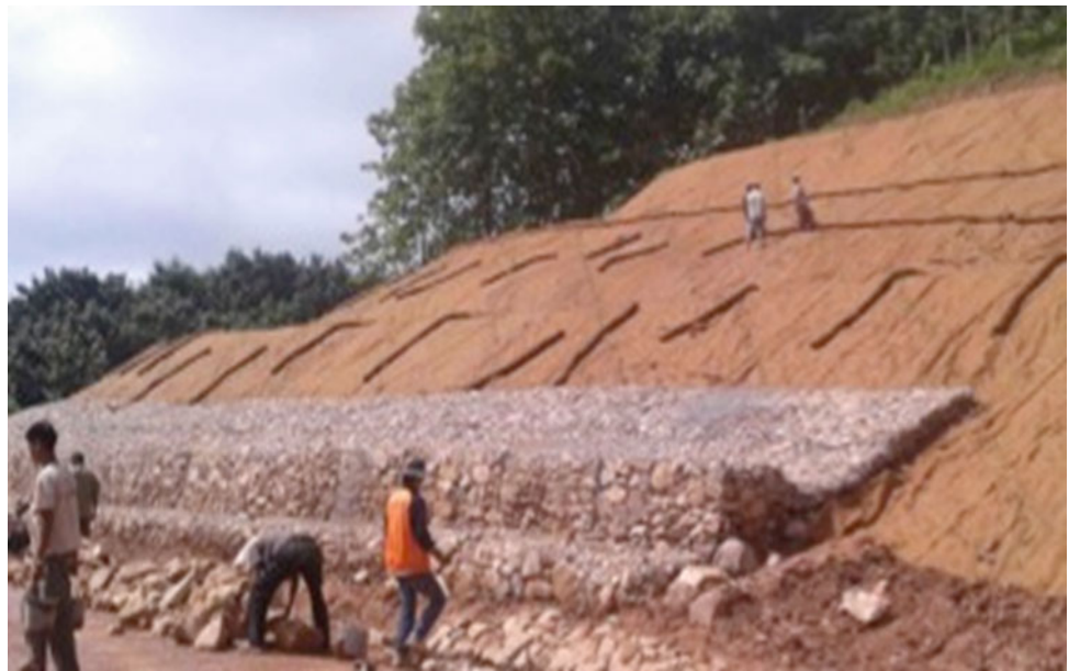
Fig. 7 Landslide mitigation, Lao PDR
