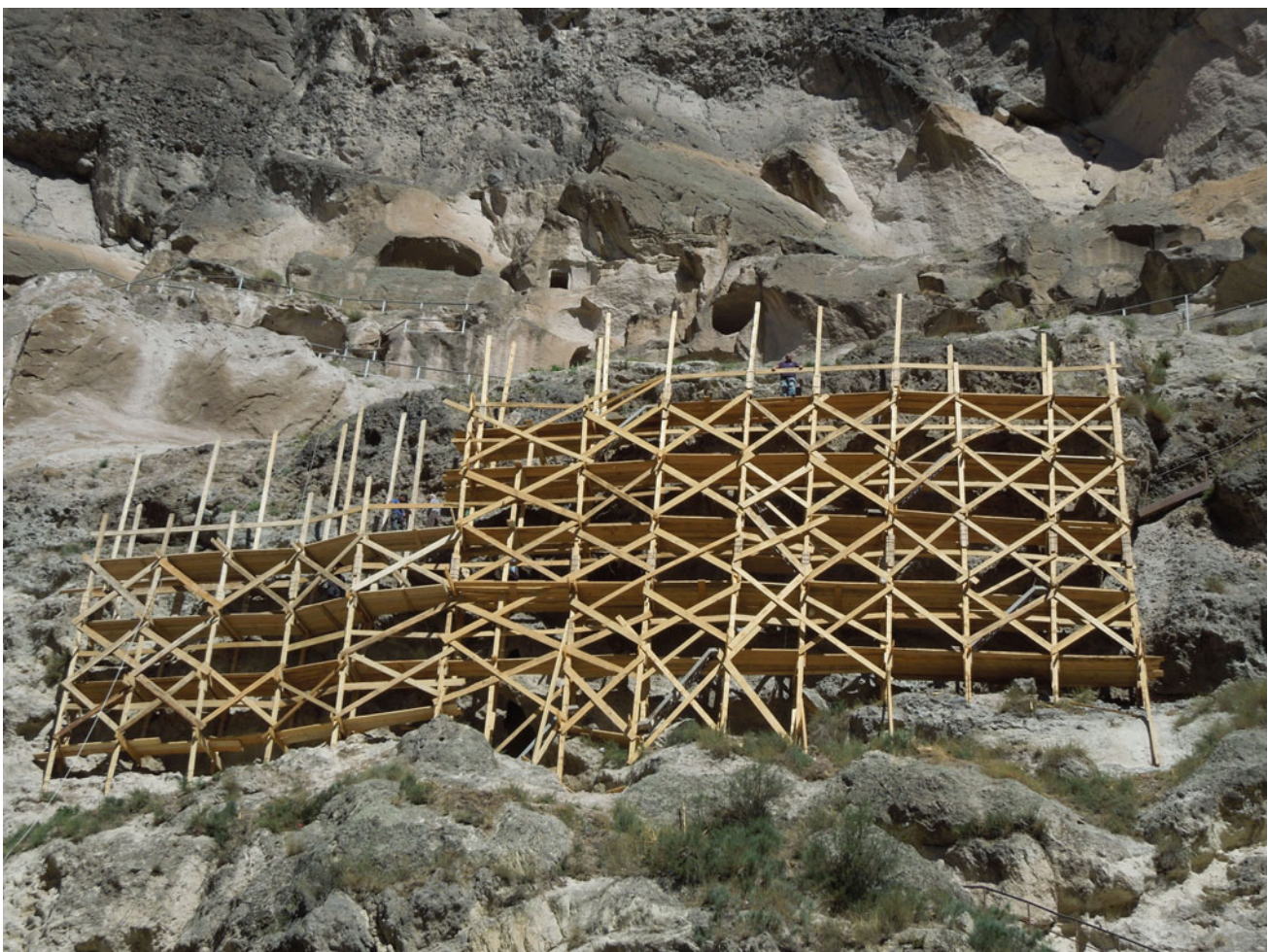
Fig. 30 The wood scaffolding realised in Vardzia
