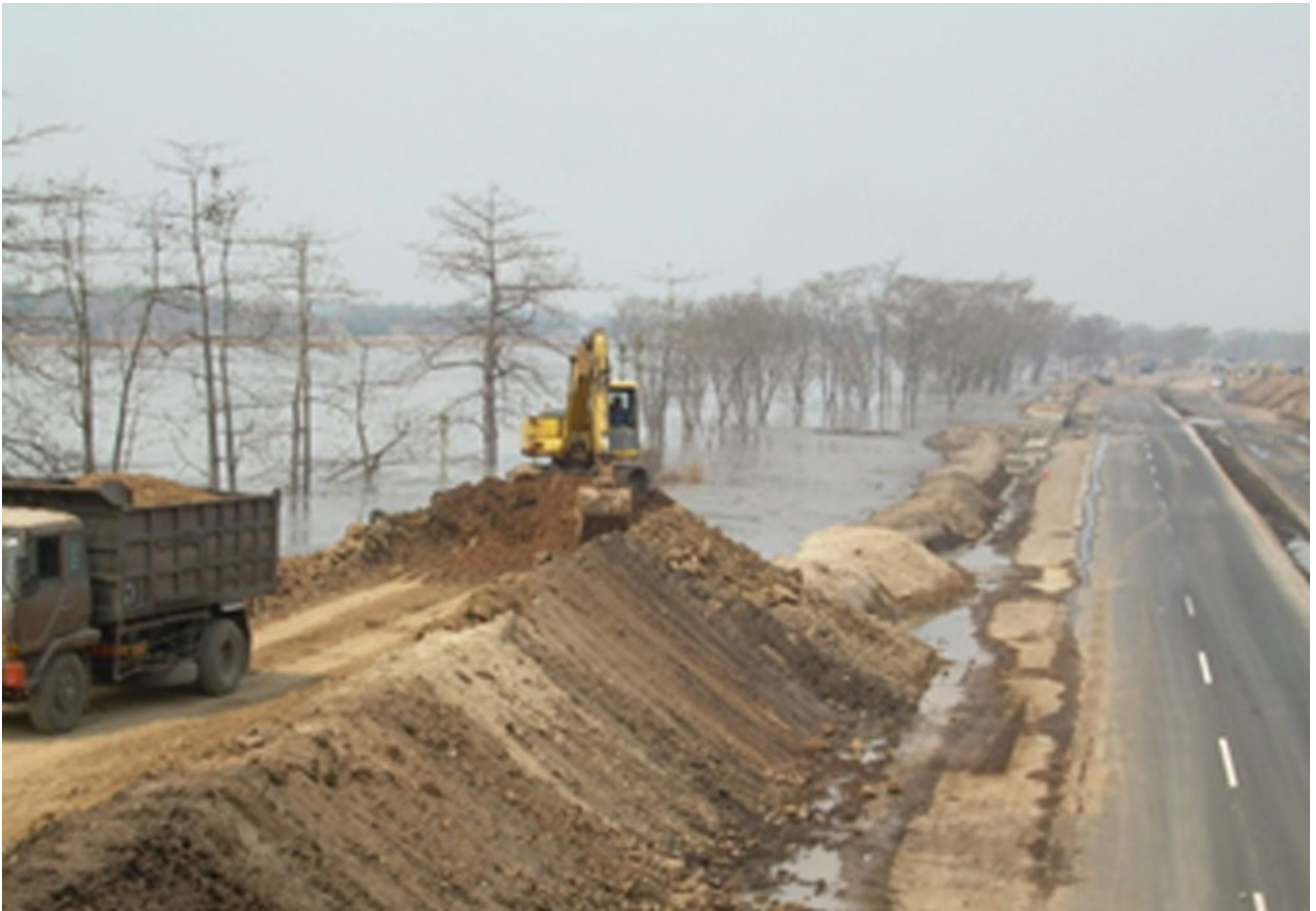
Fig. 21 Construction of permanent dykes (BPLS 2007)
