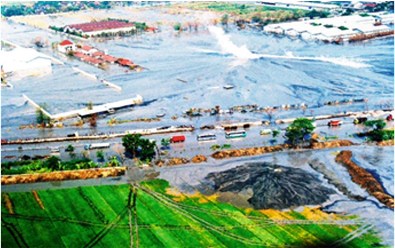
Fig. 11 Damage to area infrastructure (BPLS 2007)
