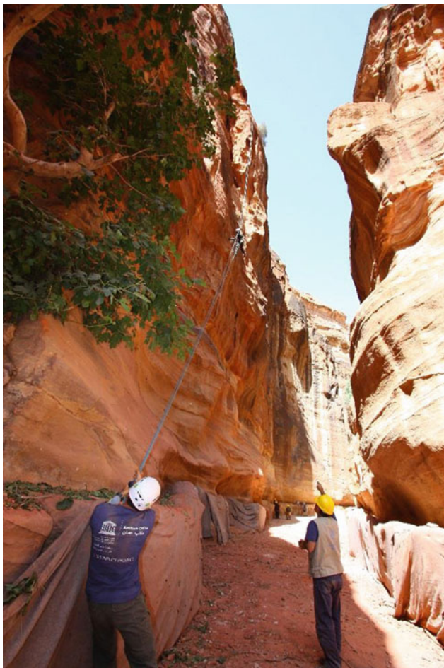
Fig. 2 Landslide risk mitigation works
