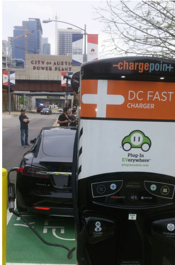
Fig. 7.4 Austin’s “Electric Drive” DCFast dual-standard station
