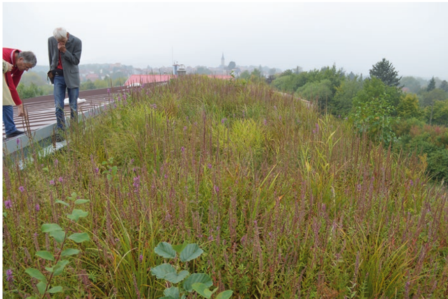
Fig. 2 Wetland roof with a surface area of 120 m 2 for the treatment of rainwater in an office building in Jena, Germany (Source: Michael Blumberg)
