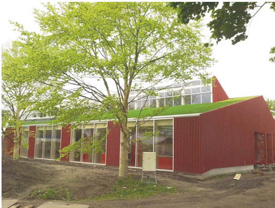
Fig. 3 A 300 m 2 constructed wetland for domestic wastewater treatment on a rooftop in the Netherlands. A portion of the treated effluent is re-used for toilet flushing (Source: Frank van Dien, ECOFYT)
