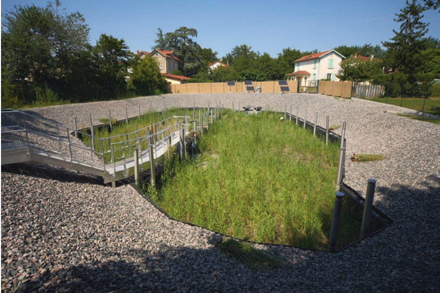
Fig. 4 The Marcy Etoile constructed wetland for combined sewer overflow treatment in Lyon, France (Source: Stephane Troesch, EpurNature)
