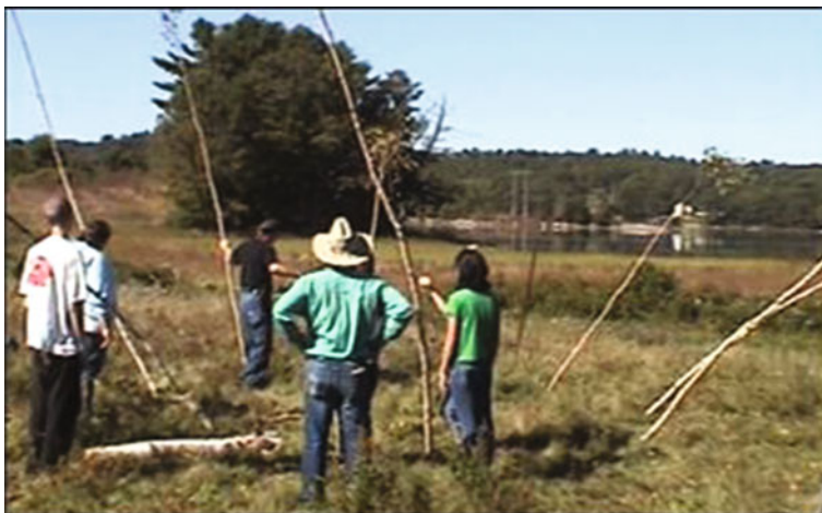
Fig. 11.7 Demonstrating how bend lodge pole toward center. Source Personal file
