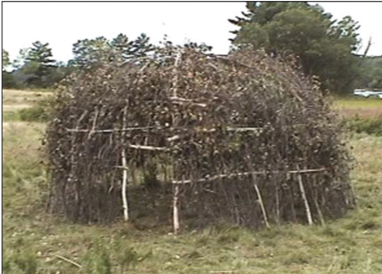
Fig. 11.11 First layer of covering on hemispherical lodge. Source Personal file
