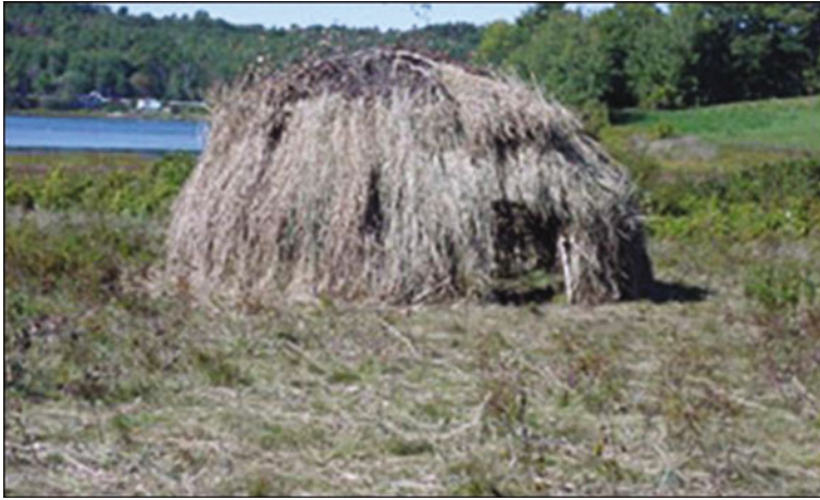
Fig. 11.12 Final layer of covering on hemispherical lodge. Source Personal file
