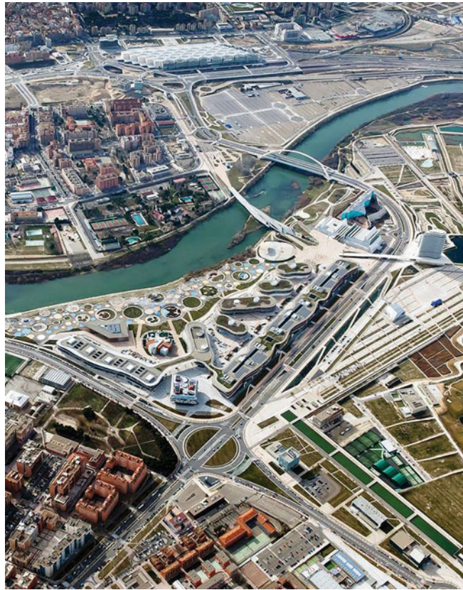
Fig. 11.9 Zaragoza, aerial photograph of the Ranillas meander which was the venue for the 2008 International Exhibition “Water and Sustainable Development”
